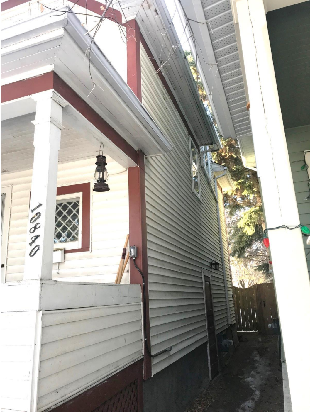
Photo #3 – Side (North) Elevation
