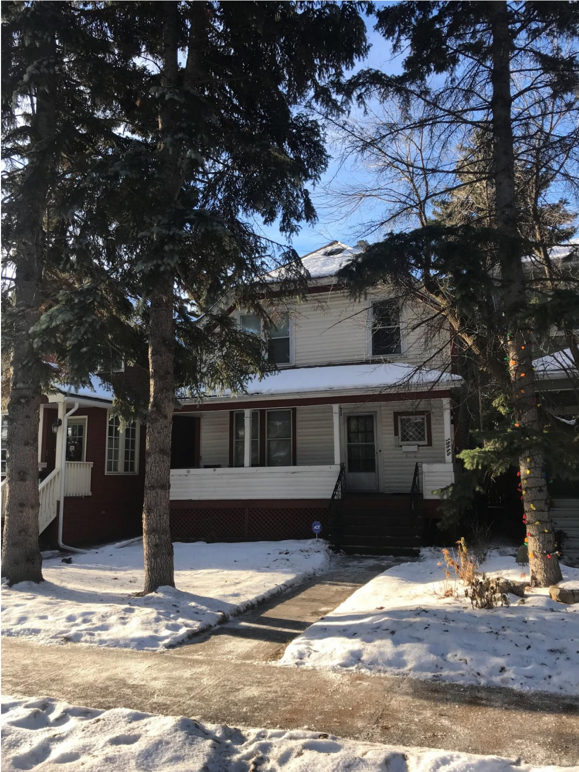
Photo #1 – Front (East) Elevation
