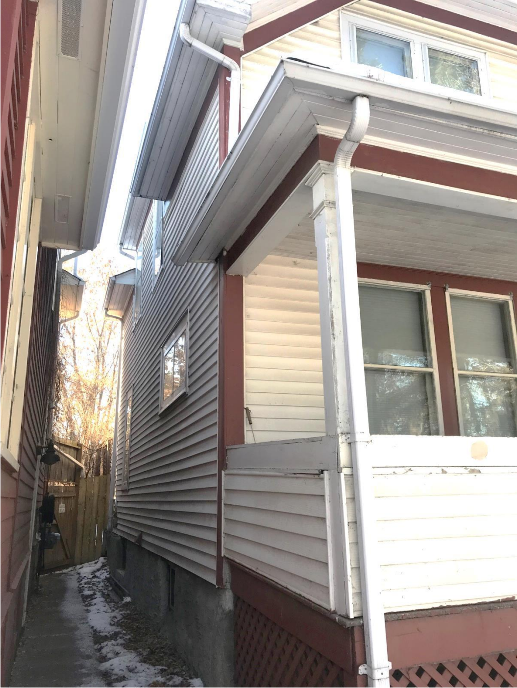
Photo #4 – Side (South) Elevation
