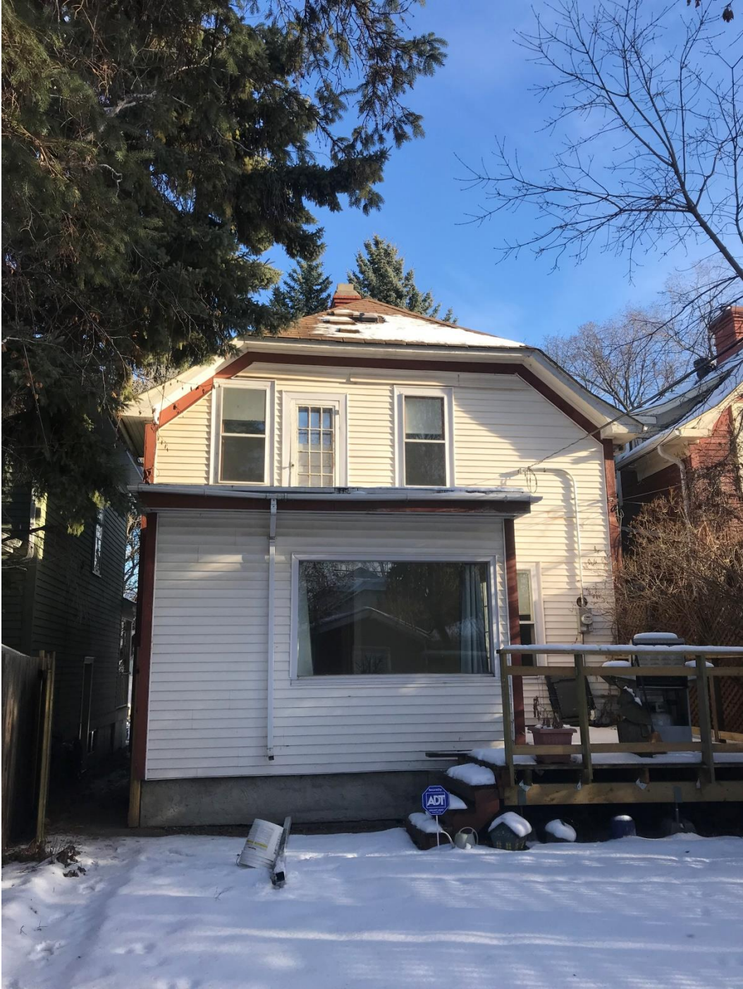
Photo #5 –Rear (West) Elevation
