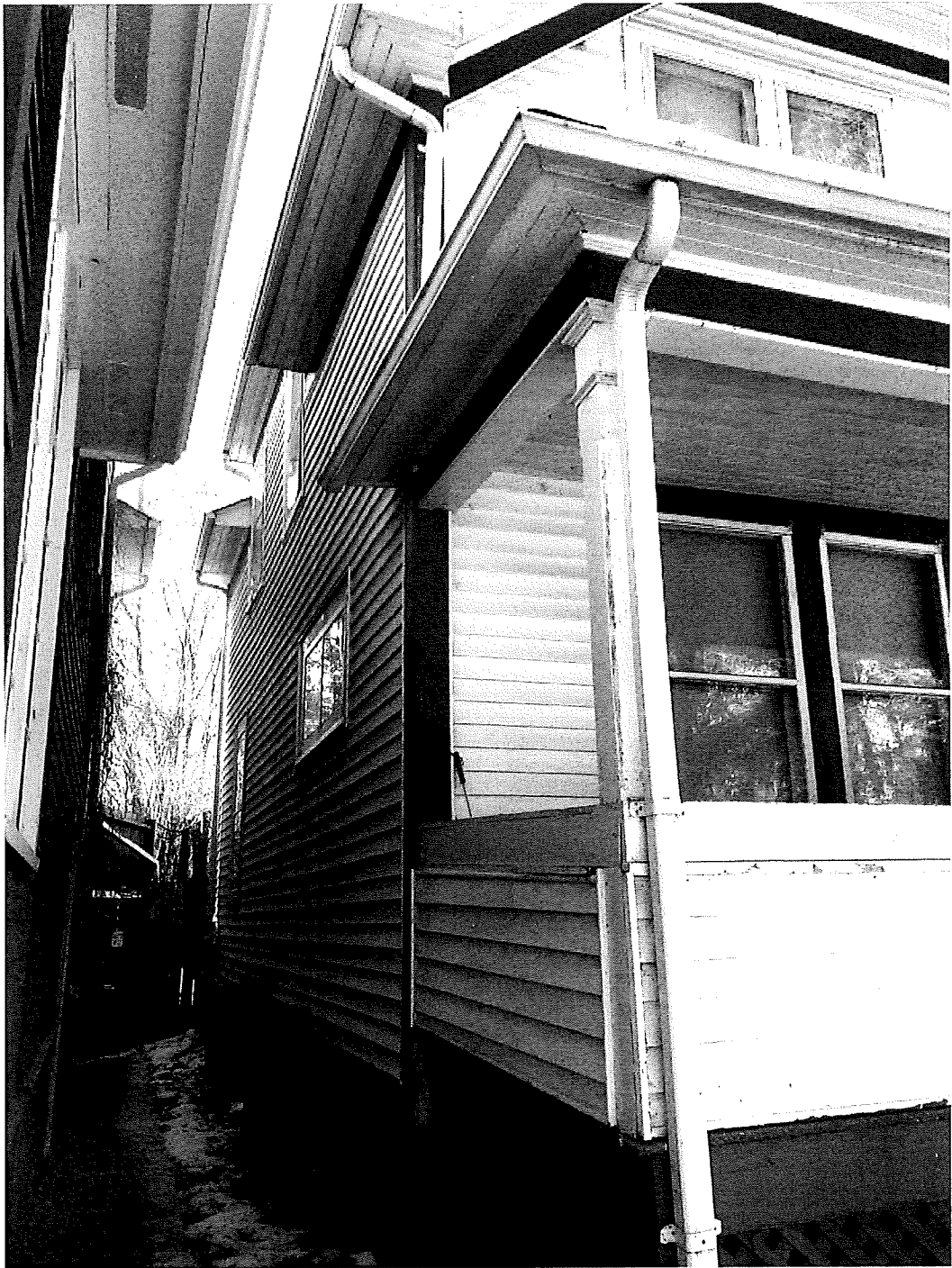
Photo #4 – Side (South) Elevation
