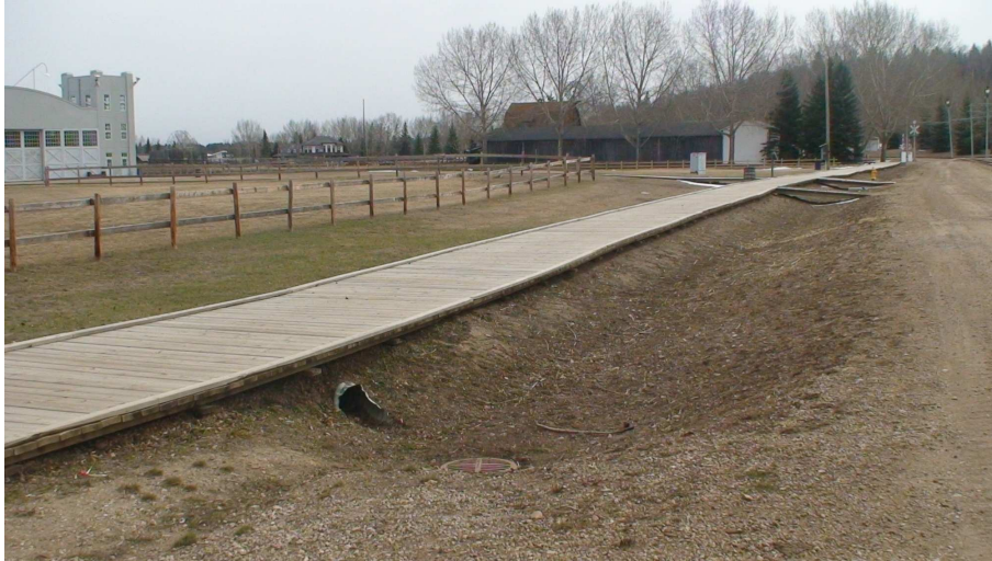
Photo #5 – Catchbasin receiving runoff from ditch and culvert
