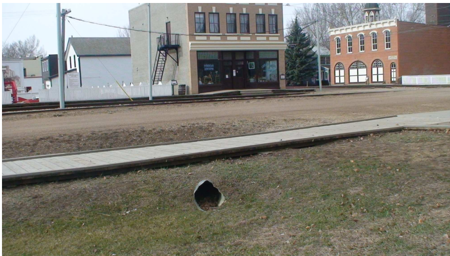
Photo #4 – Culvert at end of swale under Boardwalk
