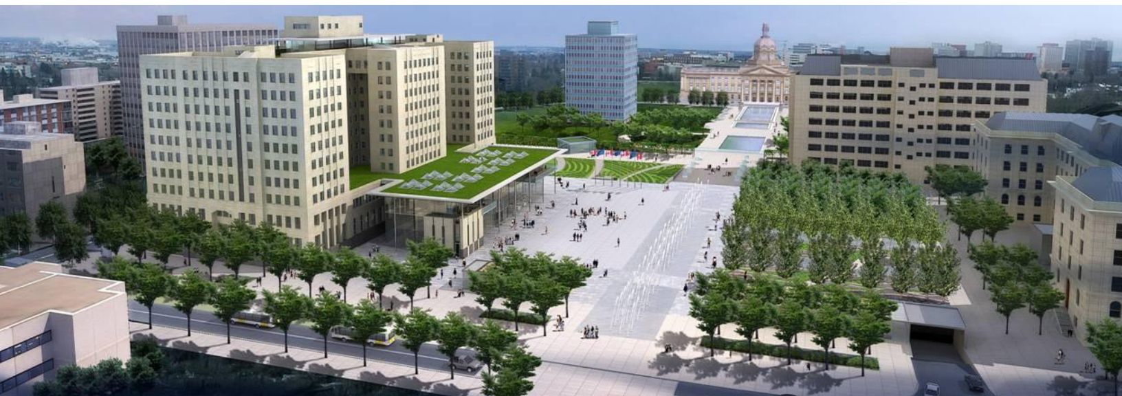
Image courtesy Carlyle + Associates
