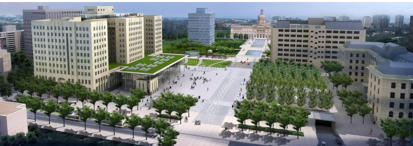
Image courtesy Carlyle + Associates
