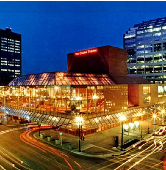
Photo courtesy Citadel Theatre
