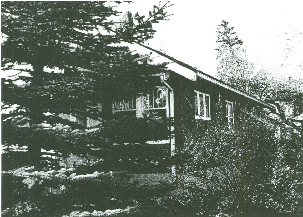
Photo #3: North East Facade
