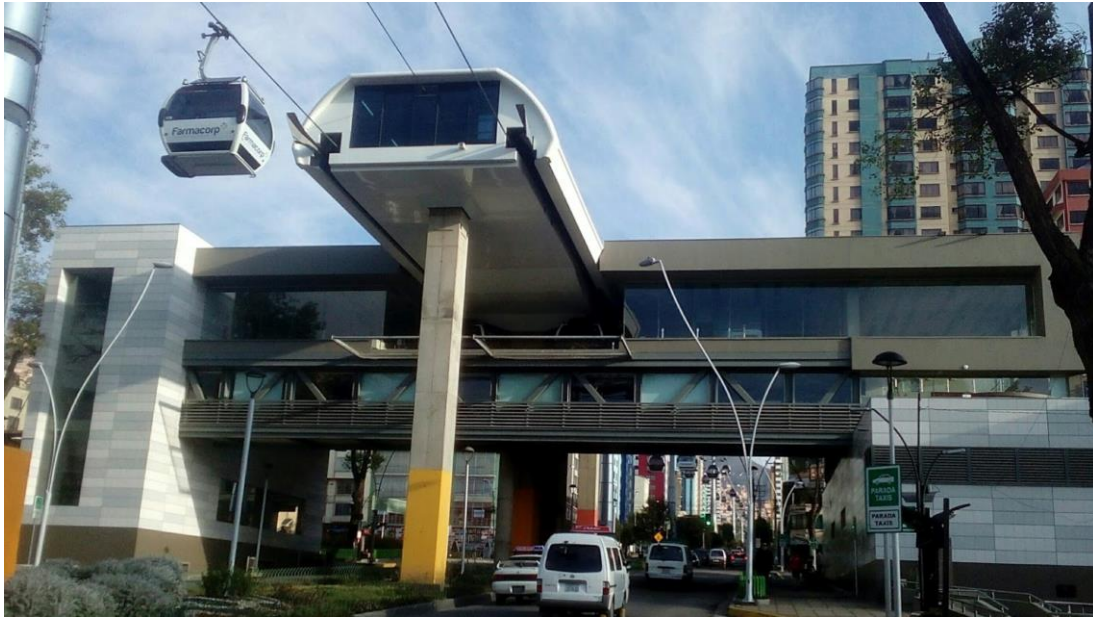
Figure 12: Mi Teleferico's White Line in La Paz, Bolivia uses a "double" Straddle station alignment with two areas of vertical circulation and a mezzanine level below platform level. It's worth noting the cantilevered design which reduces the overall bulk of the station. (Image from Google Earth)
