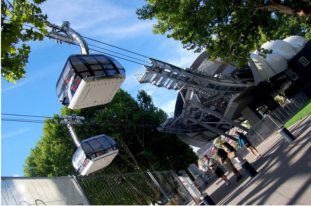
Figure 8: Koblenz Rheinseilbahn uses Simple At-Grade stations but wraps the electro-mechanical equipment in an architecturally designed membrane. (Image by Steven Dale)
