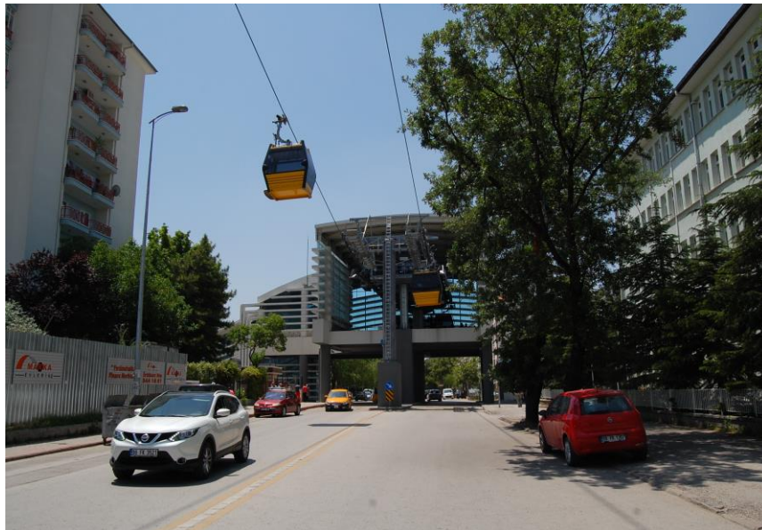
Figure 11: The Yenimahalle Teleferik in Ankara, Turkey makes extensive use of Straddle Stations. (Image by Steven Dale)
