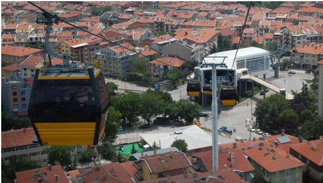
Figure 13: The Yenimahalle Teleferik in Ankara, Turkey has the only known cable car whose station is located in the middle of a roundabout. Note the pedestrian bridge leading across traffic to the vertical circulation elements. (Image by Steven Dale)
