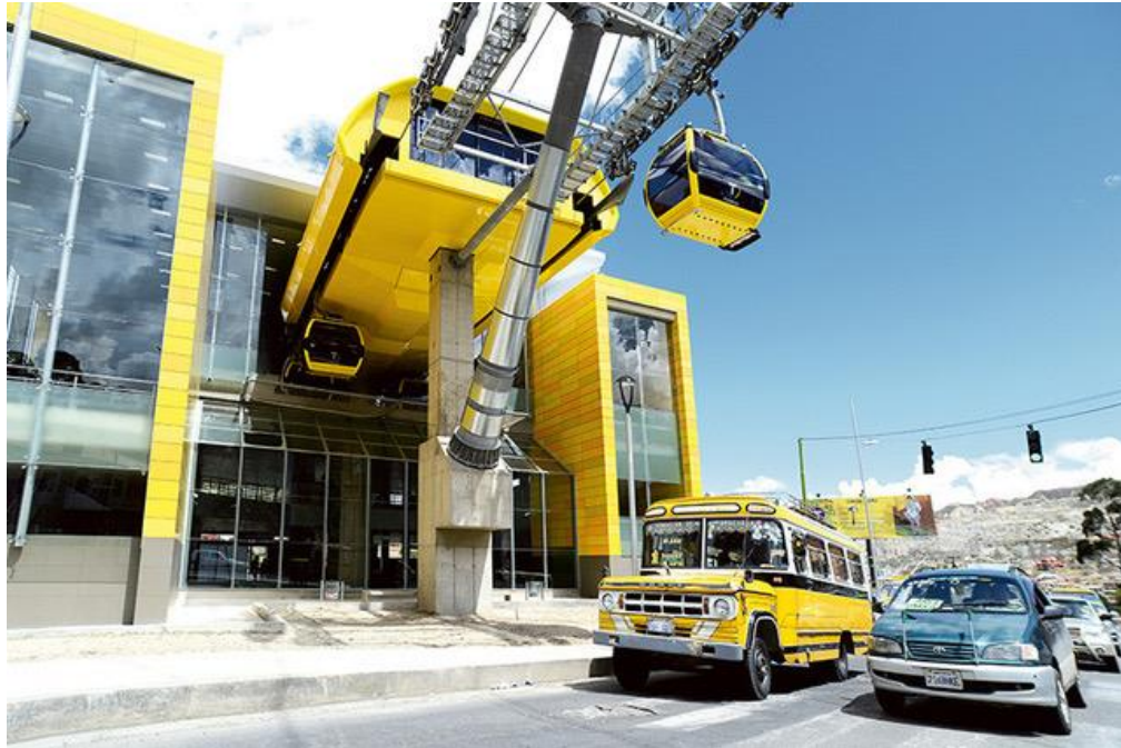
Figure 4: Mi Teleferico Cantilevered Station in La Paz, Bolivia. (Image by Doppelmayr)
