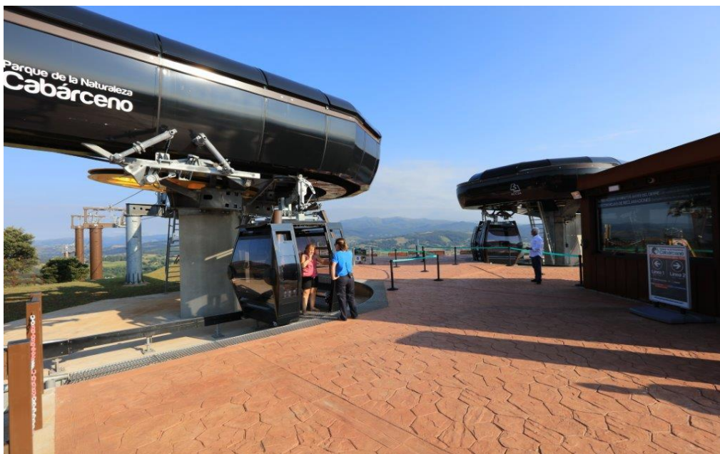
Figure 7: Cabarceno Cable Car in Spain is a Simple At-Grade station with little to no architectural considerations. (Image by Leitner Ropeways)
