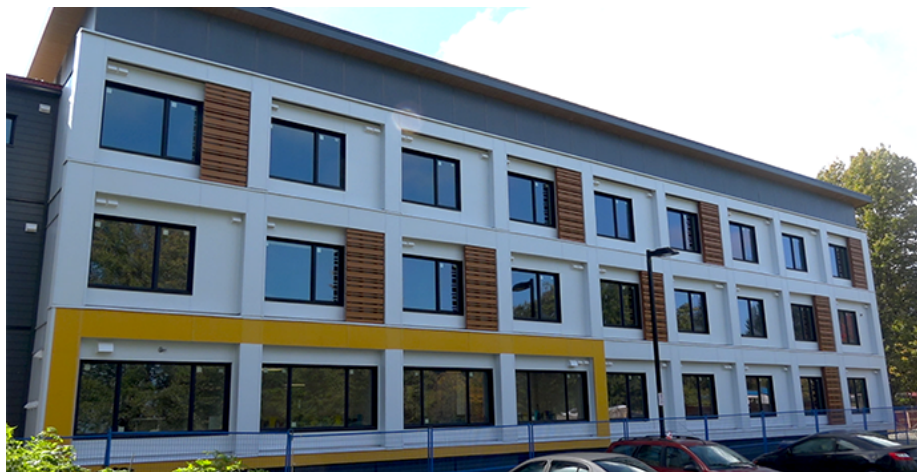
Modular permanent supportive housing in Vancouver B.C.
