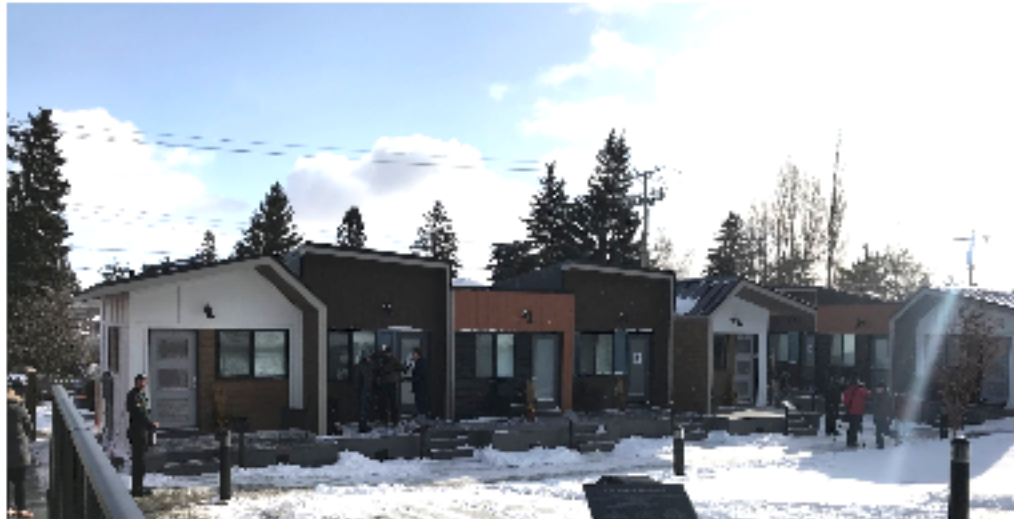
Calgary Homes for Heroes site - development completed as of November 2019.
