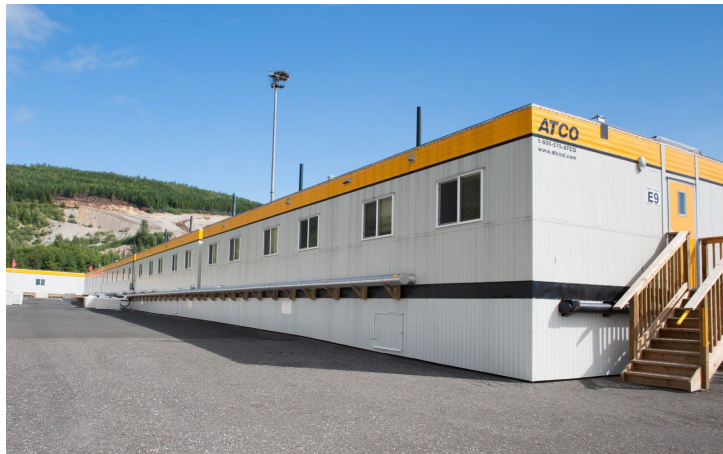
Workforce accommodations made up using several portable modules.
