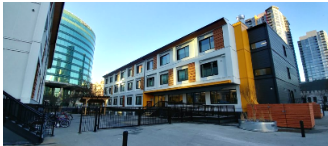
Larwill Place is a supportive housing development at 610 Cambie Street in Vancouver BC
