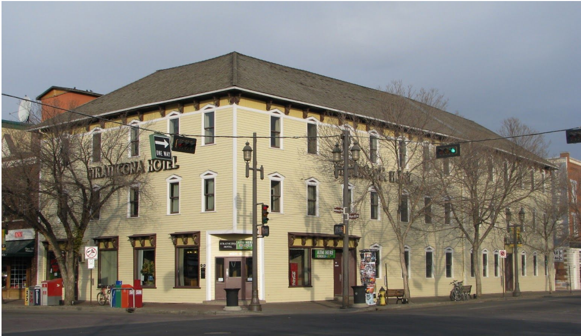
South and East Elevations (2010)
