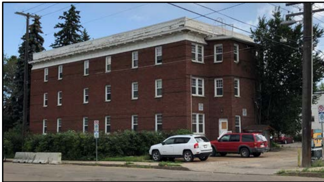
VIEW OF SITE FROM 108 STREET FACING NORTHEAST
