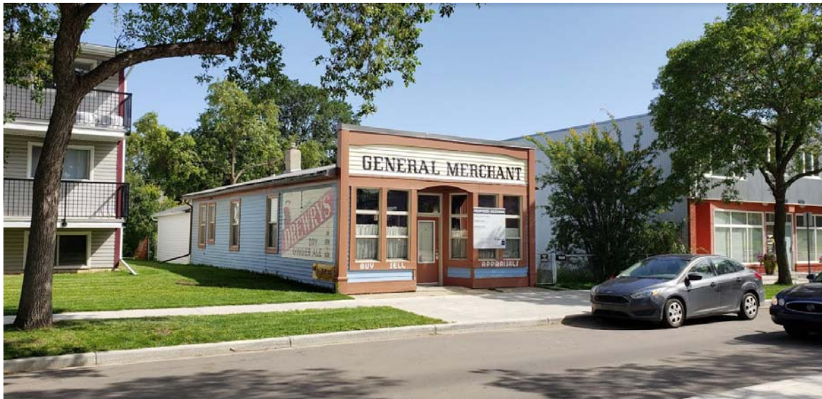
LOOKING SOUTHEAST FROM 127 STREET NW
