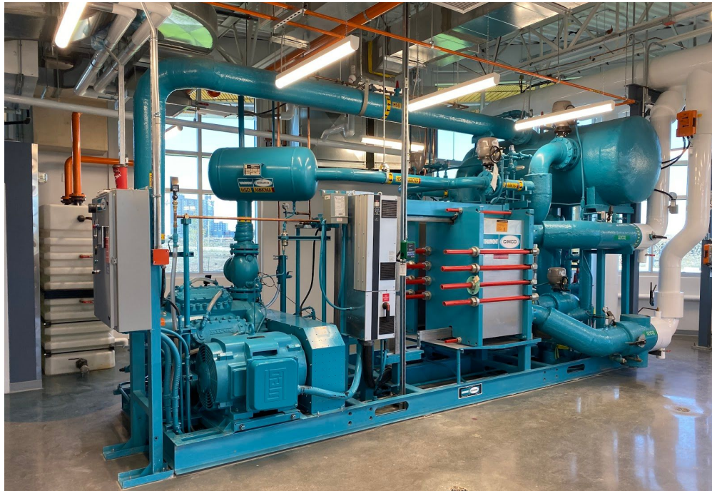
A highly energy-efficient heat pump in the Energy Centre transfers the heat from the geoechange field to the piping that runs to the community's homes.
