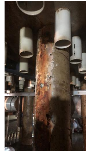
Filter Underside Structural Degradation
