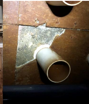
Filter Underside Structural Degradation
