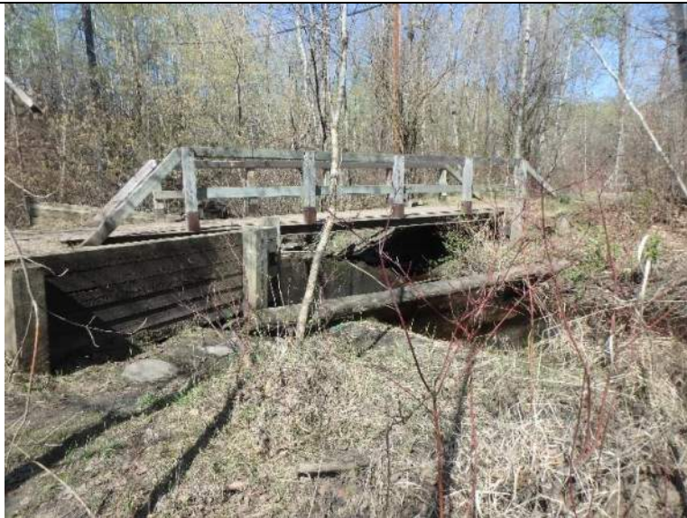
Plate 5: View downstream showing bridge B310
