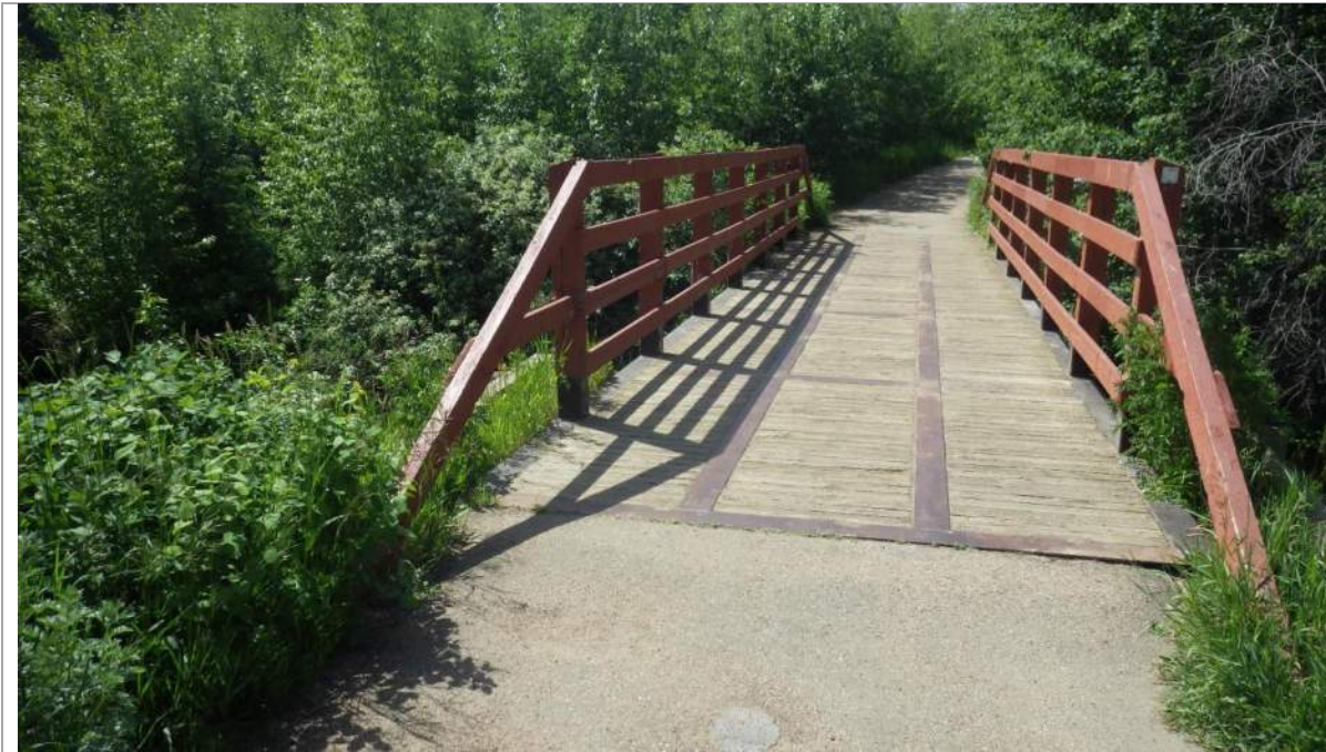
Plate 11 Bridge B314 (June 24, 2020).
