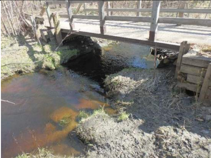
Plate 5: View upstream towards bridge B306, showing riprap already present on site.
