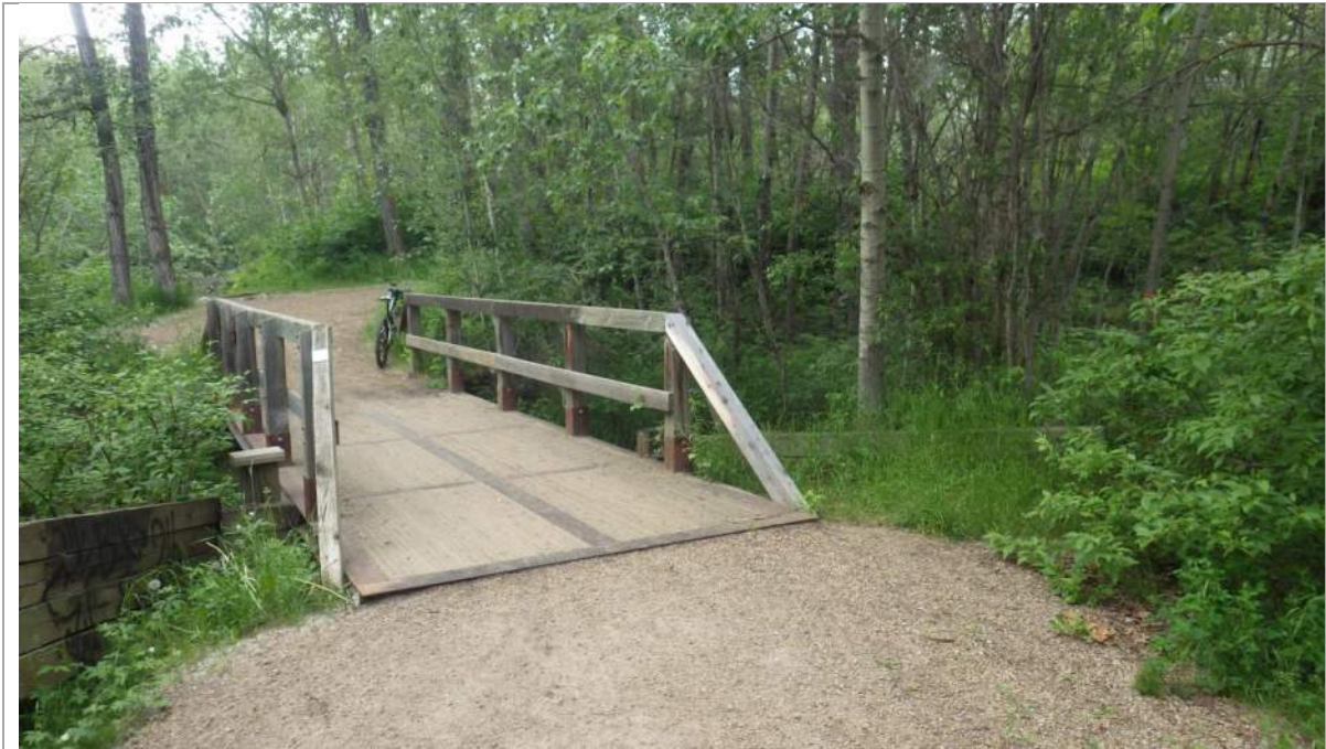
Plate 5 Bridge B308 (June 24, 2020).
