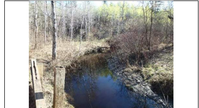
Plate 1: View upstream from bridge B304
