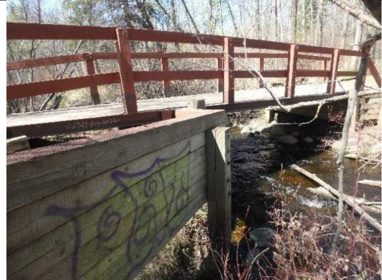
Plate 4: View across of bridge B312
