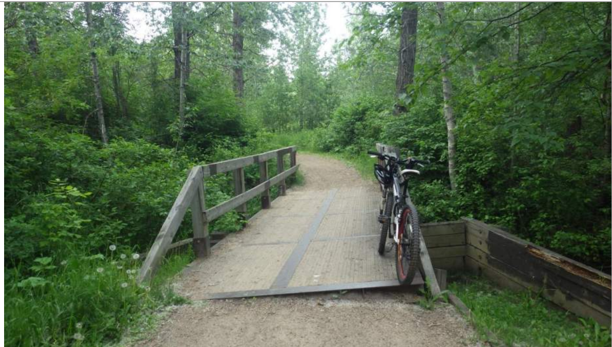
Plate 6 Bridge B309 (June 24, 2020).
