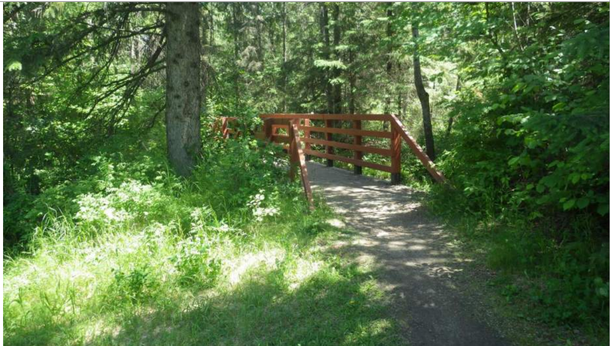
Plate 10 Bridge B313 (June 24, 2020).
