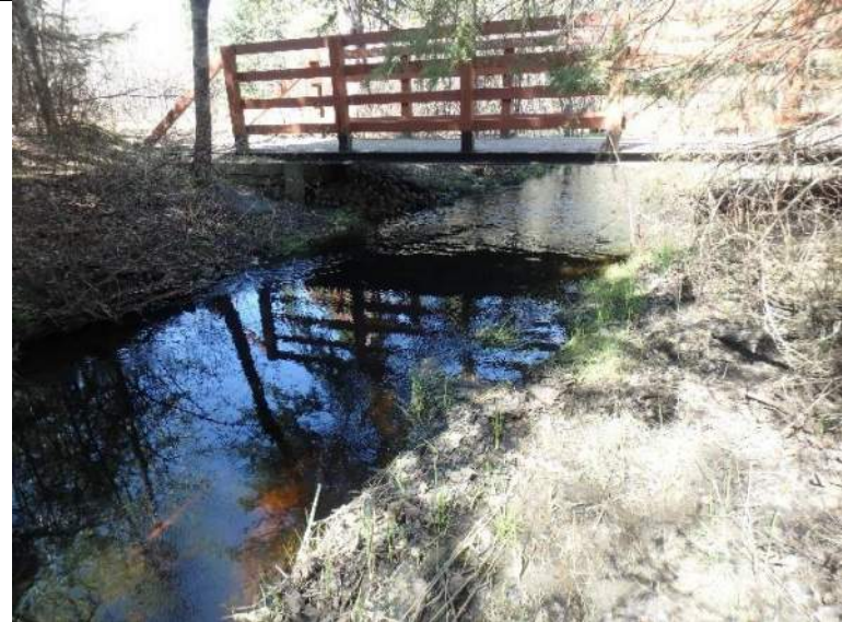
Plate 4: View downstream towards bridge B313, showing flat and riffle habitat,
