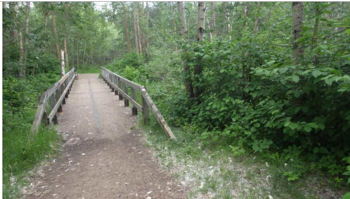
Plate 4 Bridge B307 (June 24, 2020)
