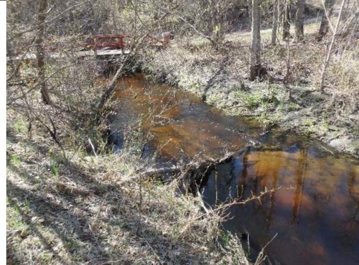
Plate 4: View downstream towards bridge B305, showing riffle habitat
