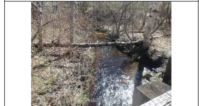
Plate 2: View downstream from bridge B309, showing large woody debris and eroded banks
