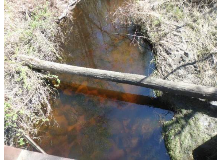
Plate 4: View upstream from bridge B310, showing rip rap presence
