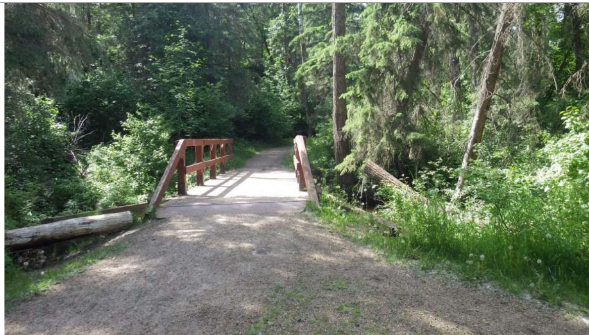
Plate 8 Bridge B311 (June 24, 2020).
