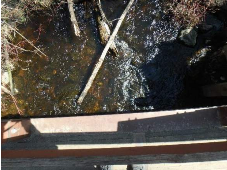
Plate 3: View showing the substrate at bridge B312
