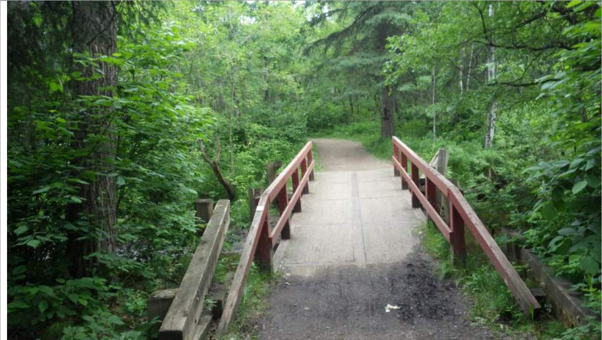
Plate 1 Bridge B304 (June 24, 2020)
