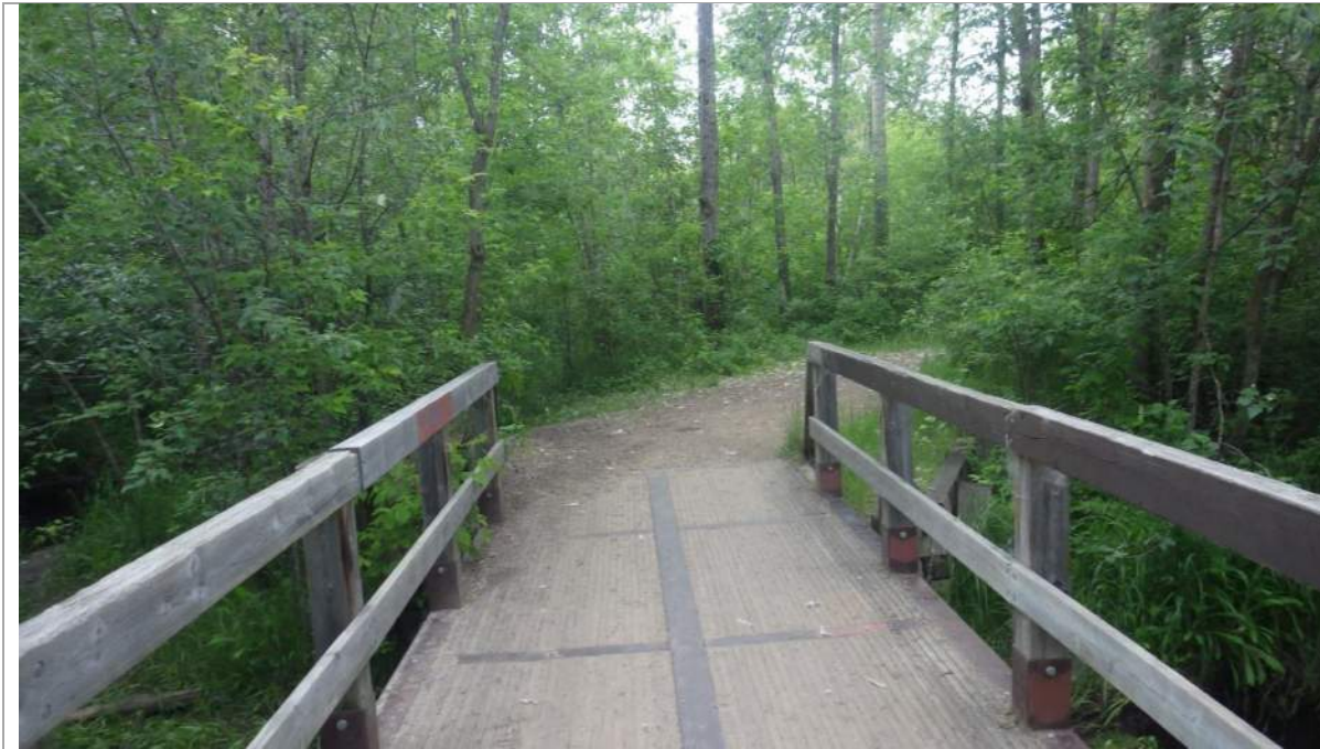
Plate 3 Bridge B306 (June 24, 2020)
