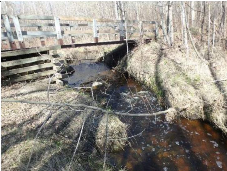
Plate 5: View upstream towards bridge B307 showing riffle downstream of bridge, and riprap present
