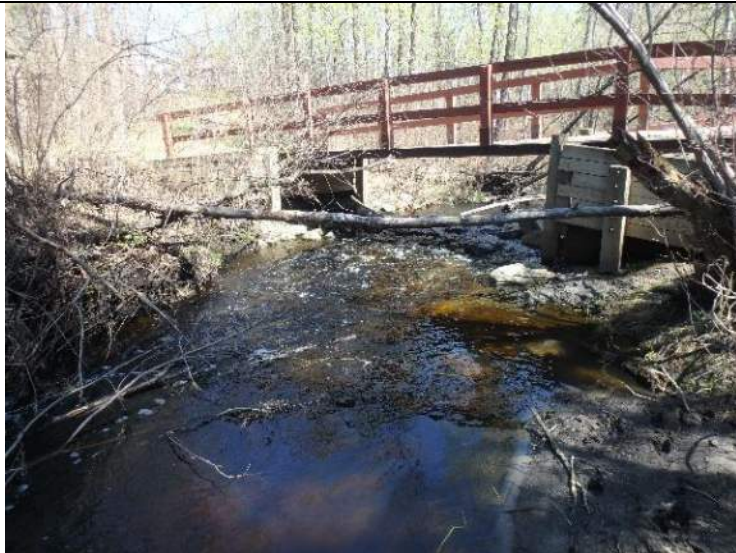
Plate 5: View upstream showing riprap present at bridge B12
