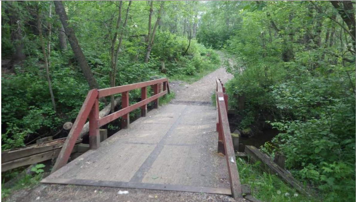
Plate 2 Bridge B305 (June 24, 2020)
