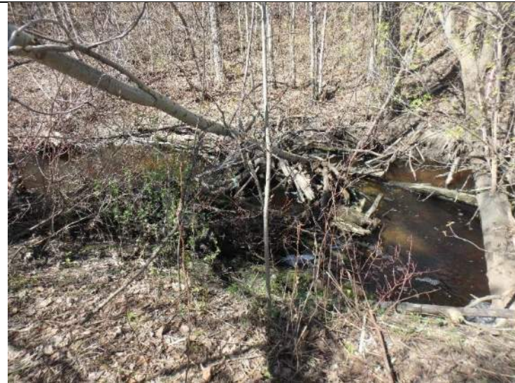
Plate 6: View showing large woody debris/dam approximately 100 m upstream of bridge B309
