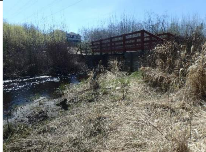
Plate 5: View downstream showing bridge B314, showing the riparian habitat
