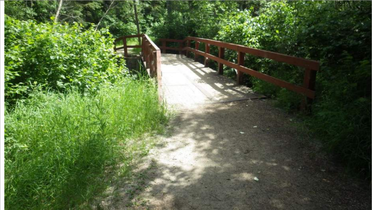
Plate 9 Bridge B312 (June 24, 2020).
