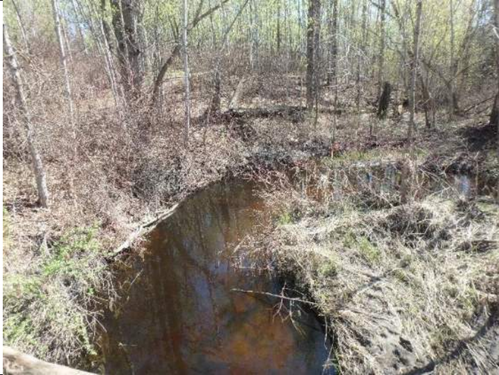
Plate 3: View upstream from bridge B310, showing backed up flows
