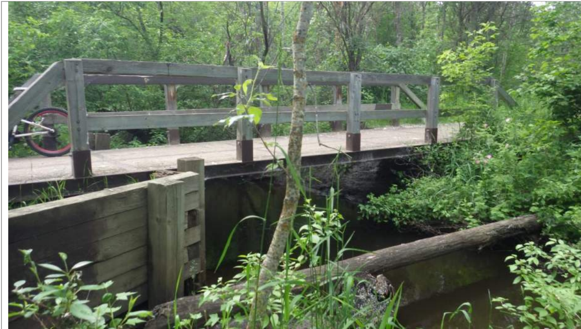
Plate 7 Bridge B310 (June 24, 2020).
