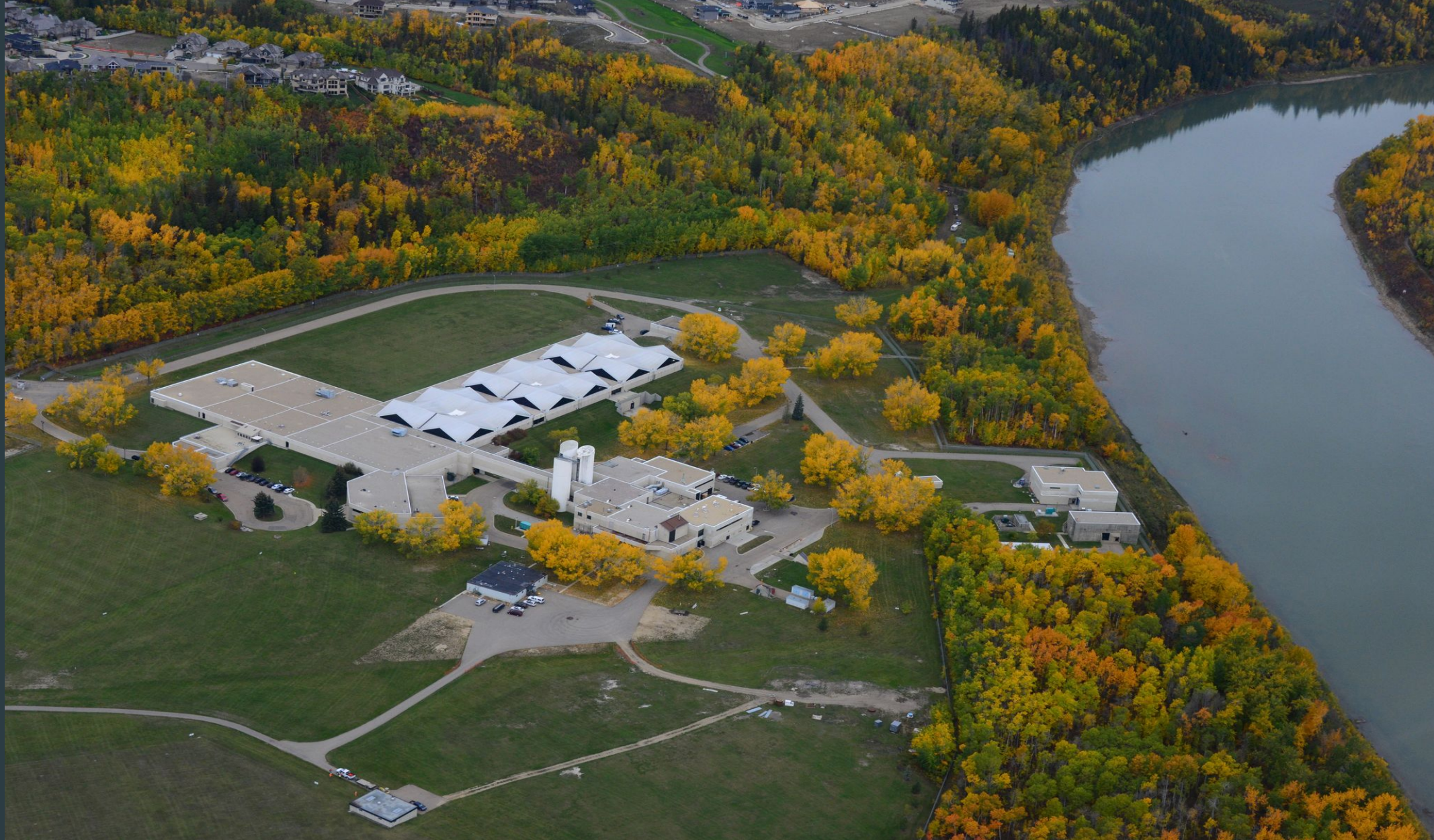
Epcor Water Treatment Plant (ca. 2019)
