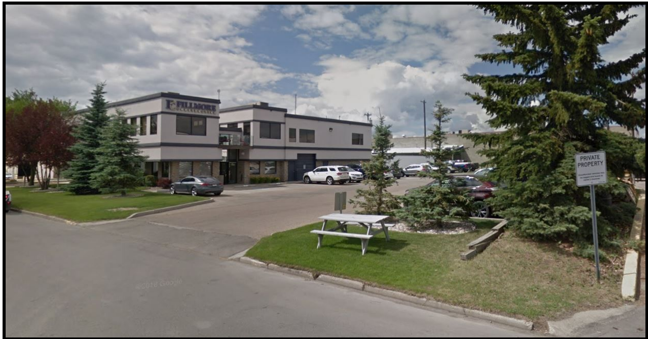
VIEW OF SITE LOOKING NW FROM 34A AVENUE NW
