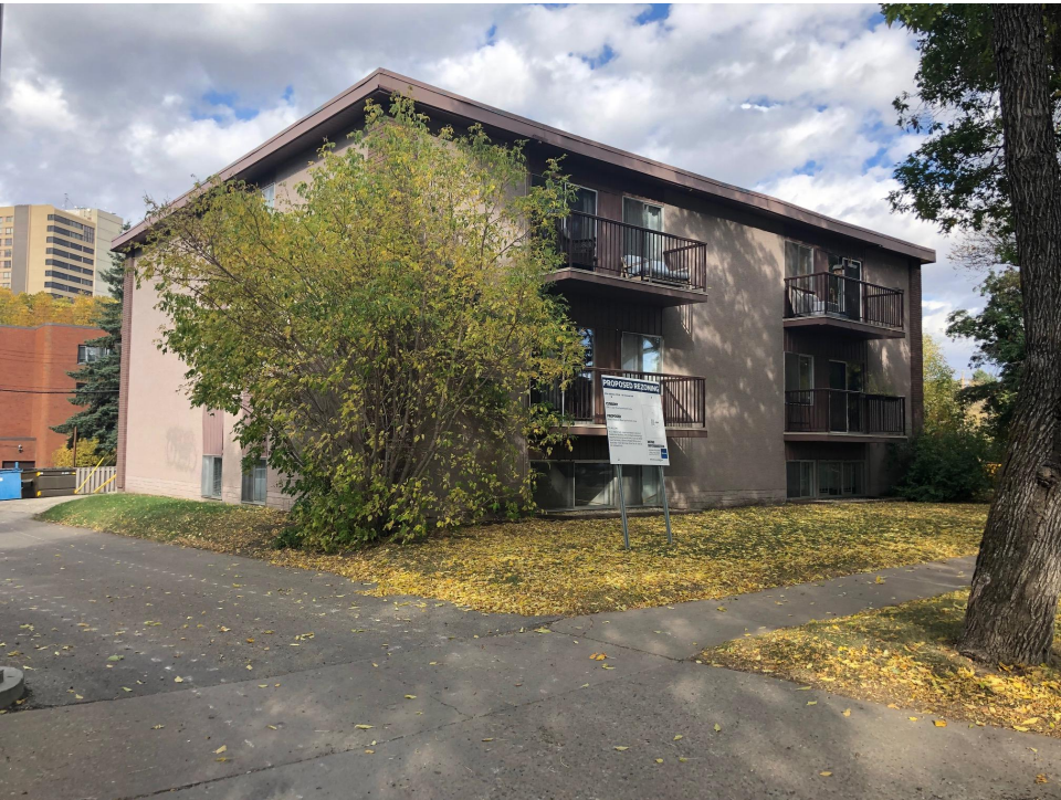
VIEW OF SITE LOOKING NORTHEAST
