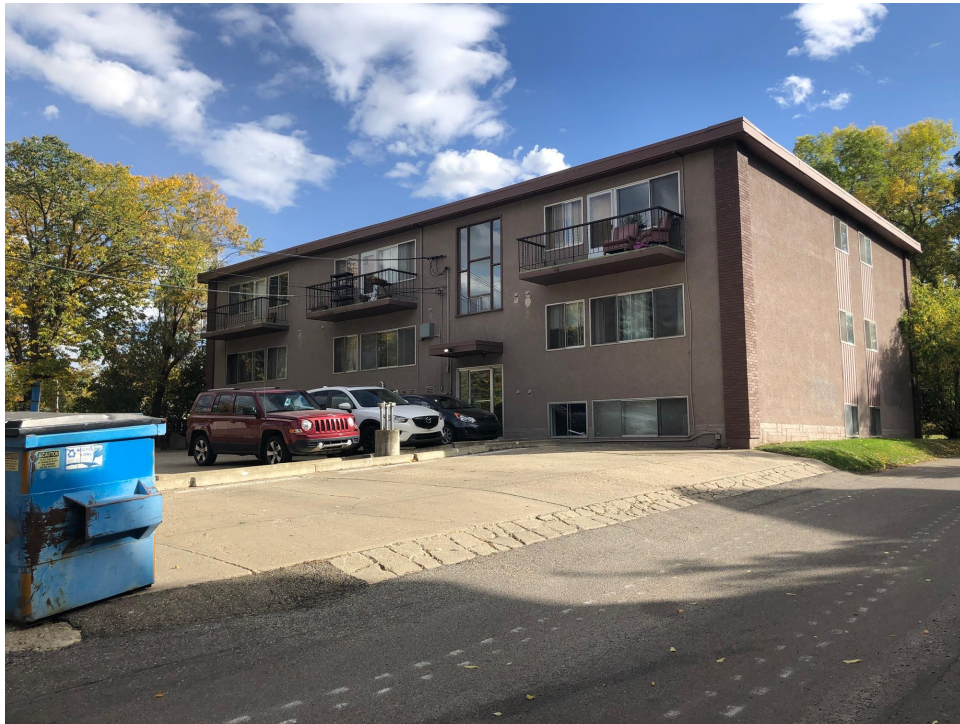
VIEW OF SITE LOOKING SOUTHEAST
