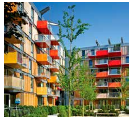
Figure 20 Medium Rise Apartments
