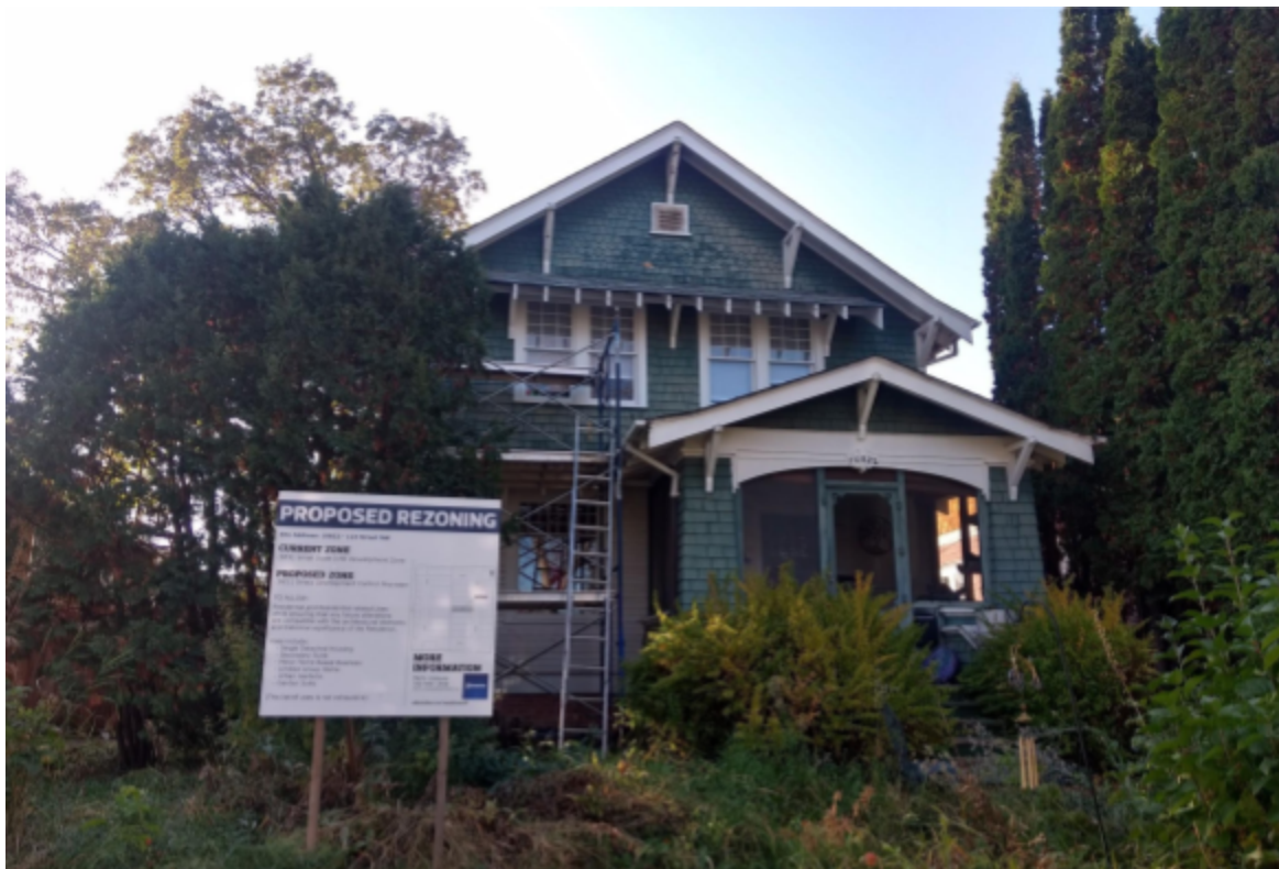
VIEW OF THE SITE FACING WEST FROM 123 STREET NW
