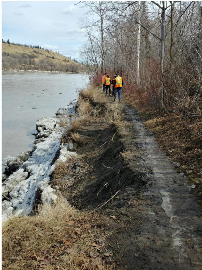
**Plate 1.1. Slumping of the south bank of the NSR along Riverside Trail (Location 1) (22 April 2020).**
