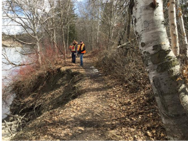
Plate 2. Slope failure of the south bank of the NSR along Riverside Trail (Location 6) (22 April 2020).
