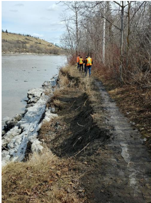
Plate 1. Slope failure of the south bank of the NSR along Riverside Trail (Location 1) (22 April 2020).
