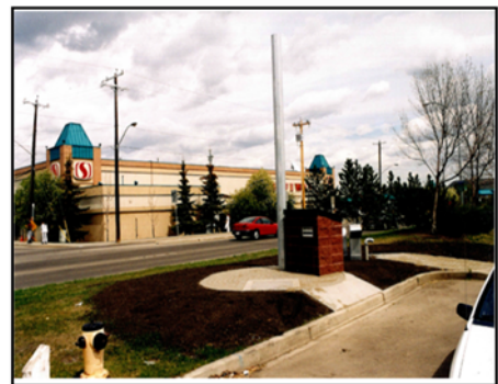
West End Odour Filter – 151 St/100 Ave
