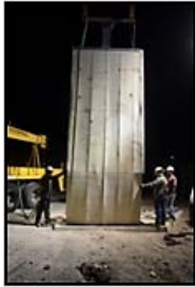
Example of an air curtain in the City of Los Angeles
