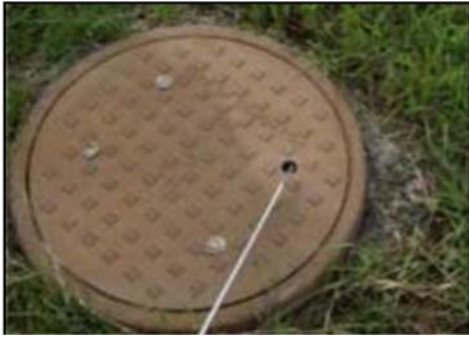
Examples of manhole pick inserts and a manhole sealing installation (ISC)
