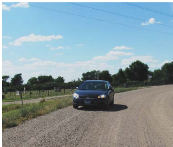
Well-shaped superelevation on a curve.
