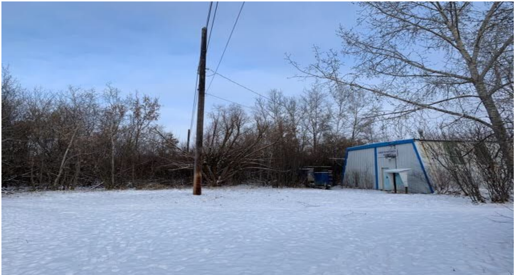
EWB Storage site at Buena Vista Park
