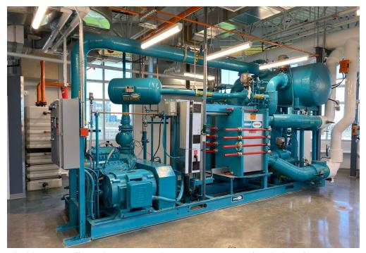
A highly energy-efficient heat pump in the Energy Centre transfers the heat from the geoexchange field to the piping that runs to the community's homes.
