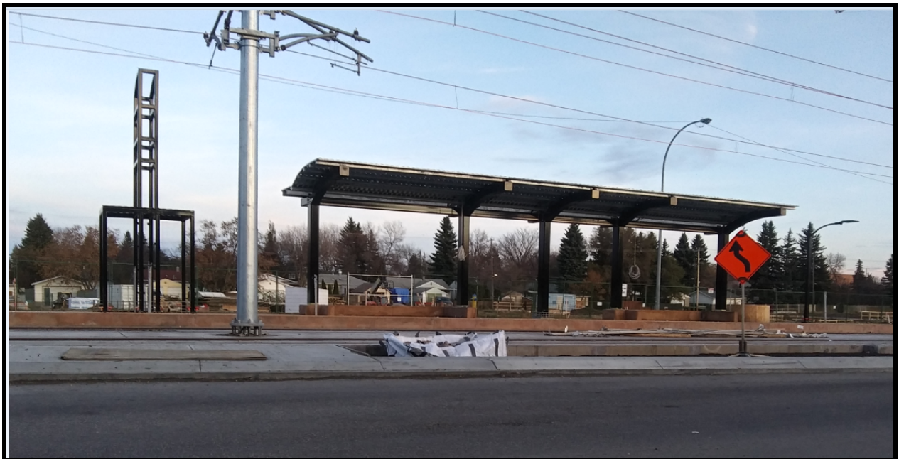
VIEW OF LRT STATION FROM 85 STREET NW
