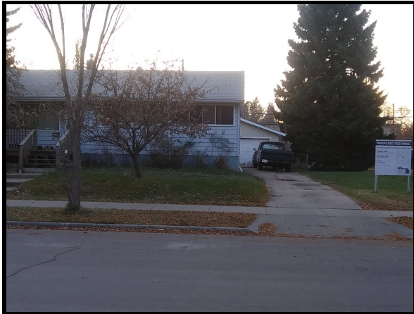
VIEW OF SITES FROM 83 STREET NW
