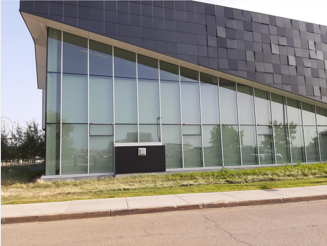
Rear of library – facing north
