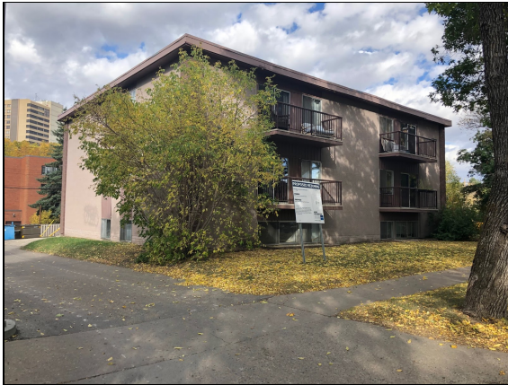
VIEW OF SITE LOOKING NORTHEAST
