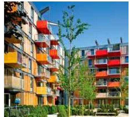
Figure 20 Medium Rise Apartments
