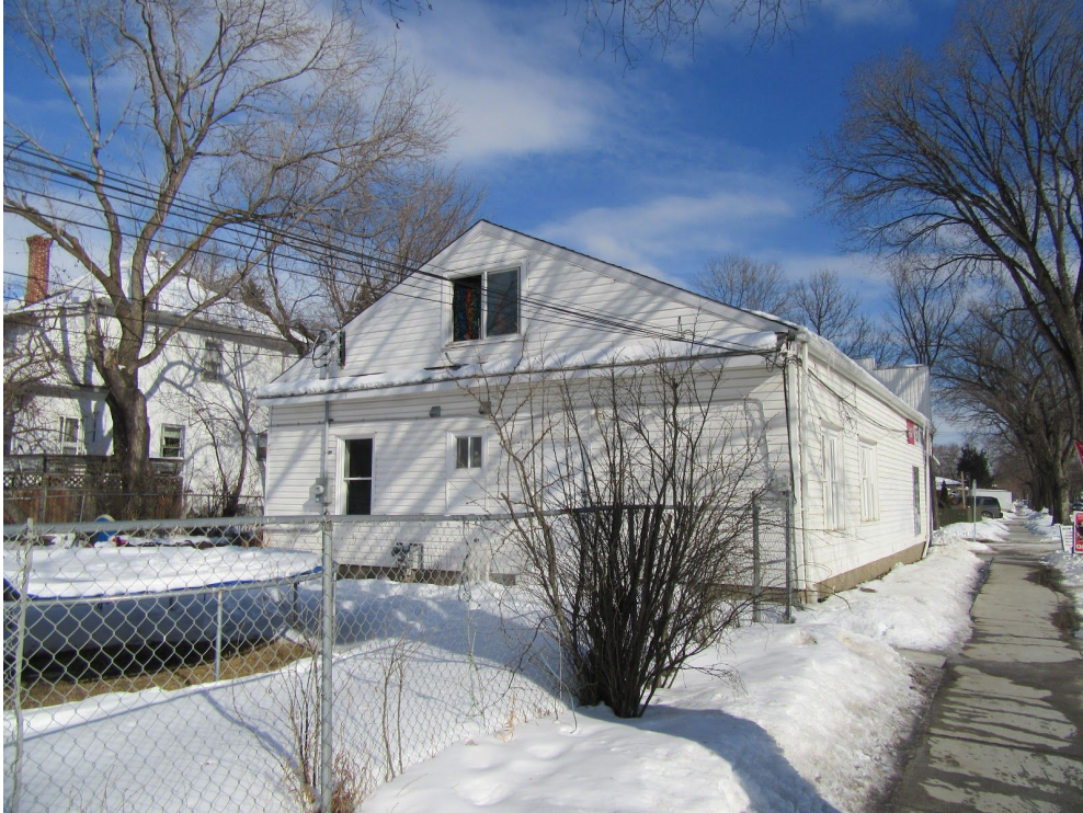
West elevation, viewed from 122 Avenue NW
