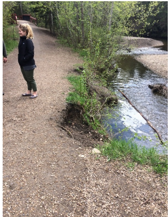
Figure 10 Site 3 looking south with Bridge 207 in the background
