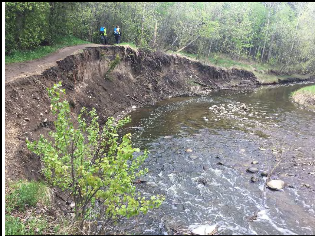
Photo 1: Site 1; eroded right bank of Mill Creek (facing east)
