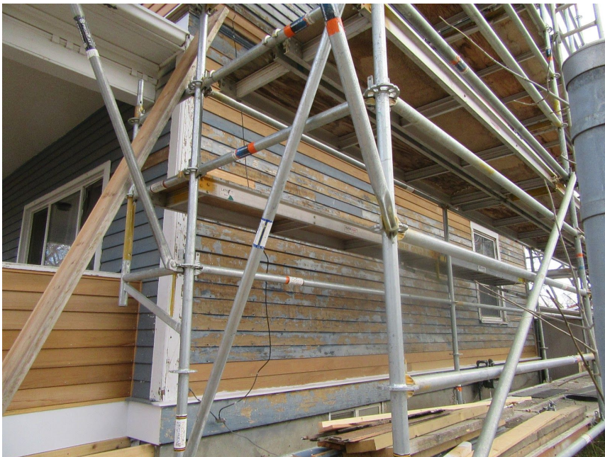
View of south elevation, showing restoration of existing wood cladding.
