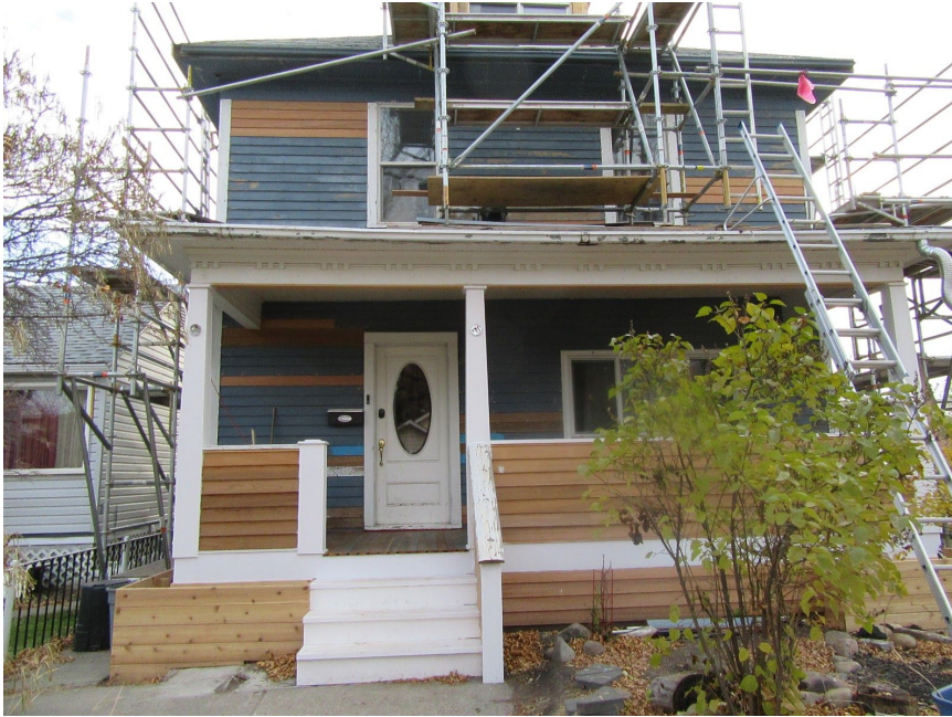
View of west (front) elevation, showing restoration of existing wood cladding.
