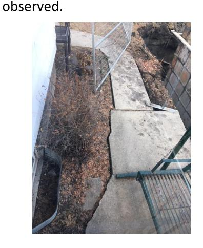
Sloughing of excavation walls is also observed.
