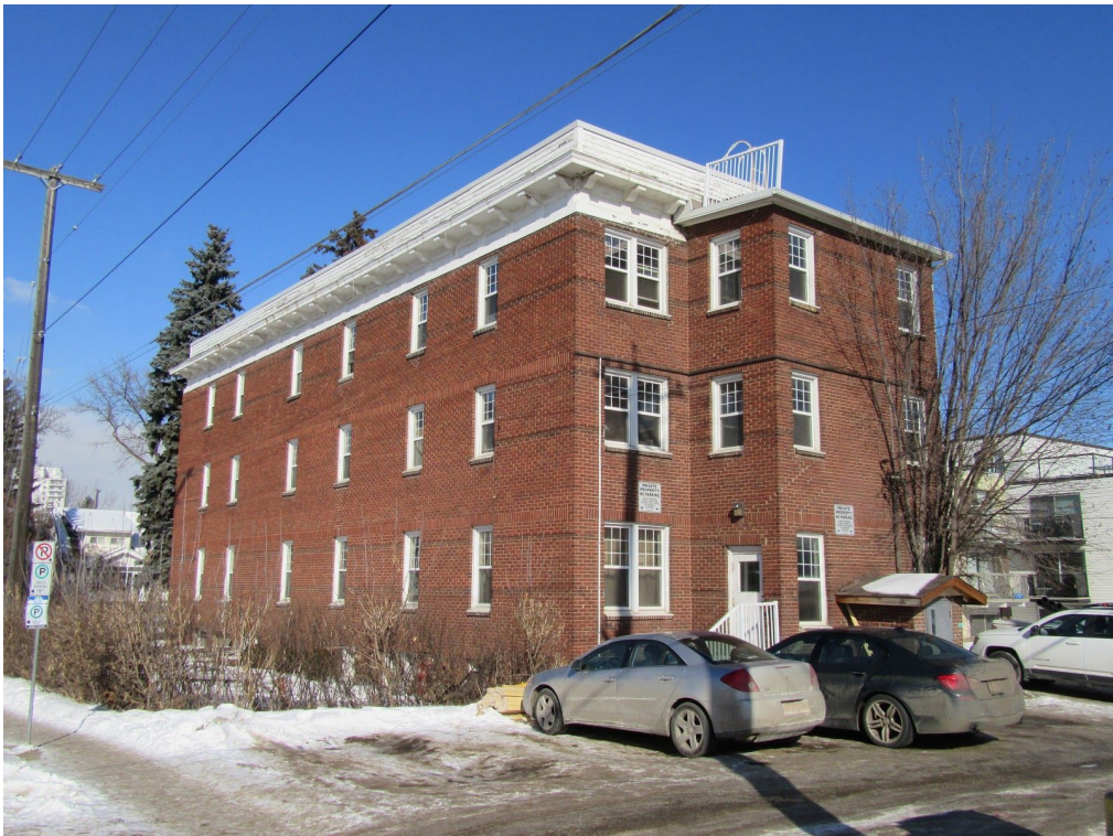
West and south (rear) elevations, viewed from 108 Street NW (the south elevation is not included in the designation)
