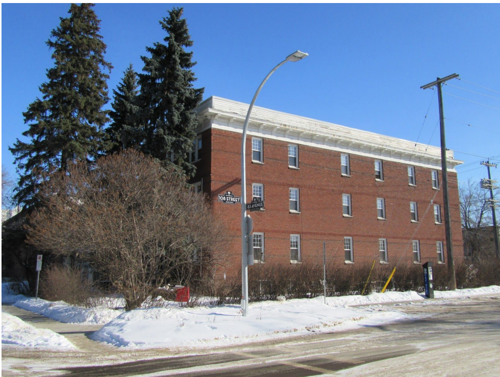
North and west elevations, view from 108 Street NW
