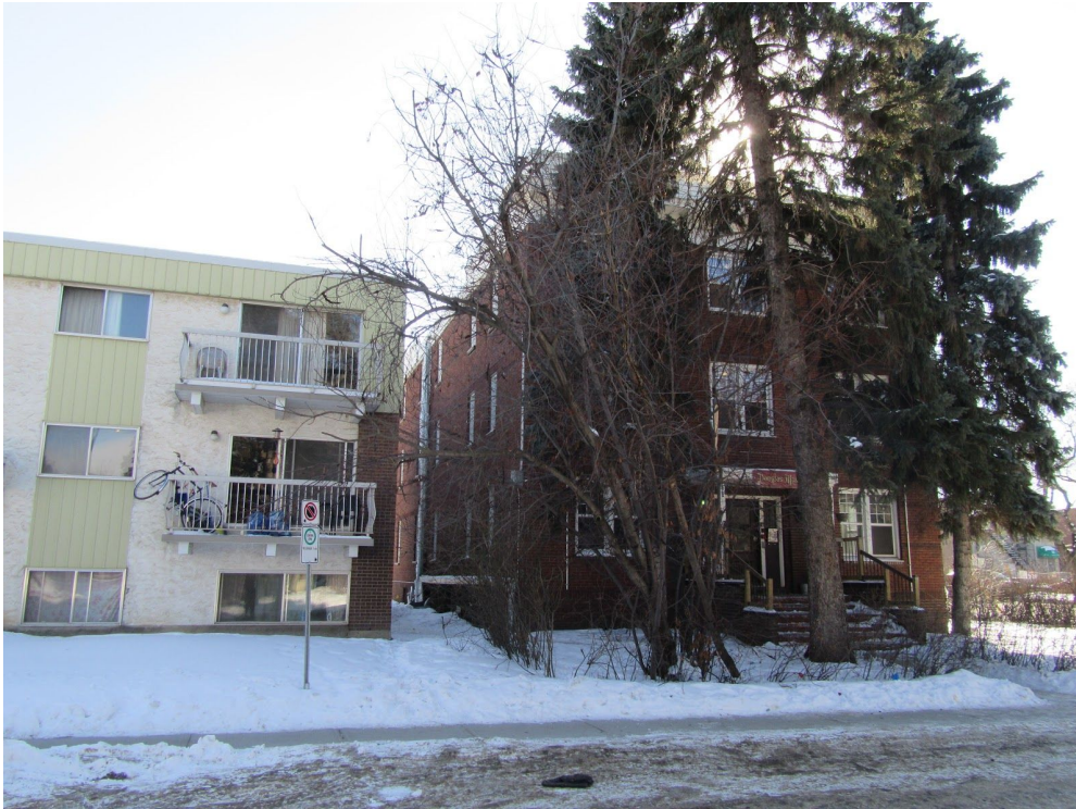
East and north elevations, viewed from 83 Avenue NW
