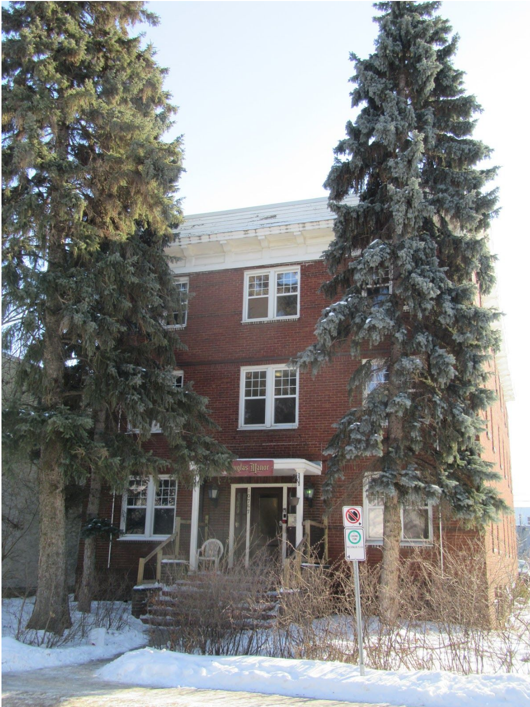
North (front) elevation, viewed from 83 Avenue NW
