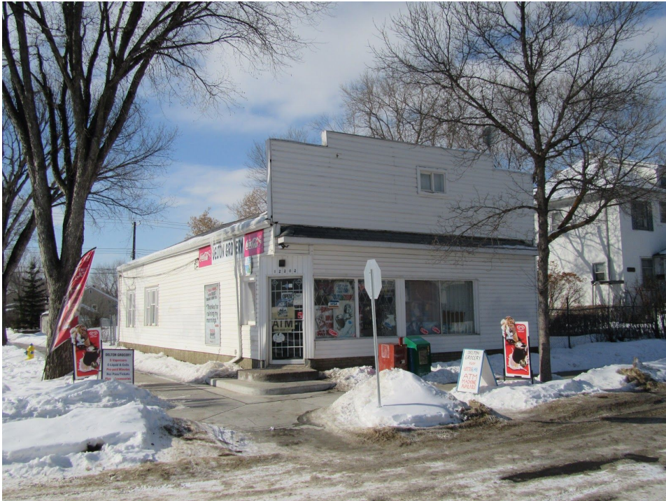
East (front) and south elevations, viewed from 122 Avenue NW
