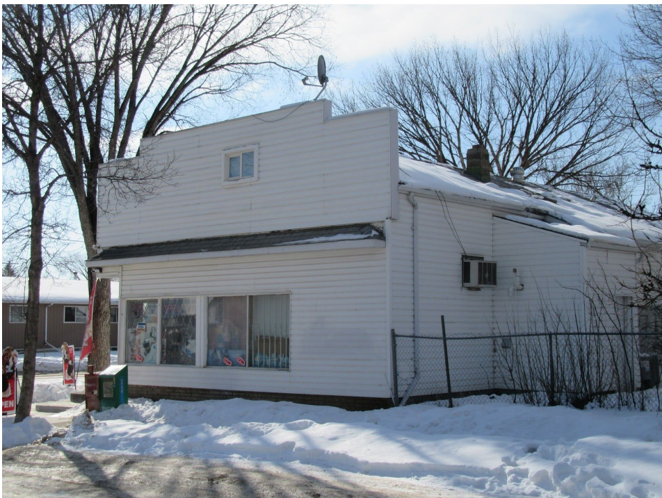
East (front) and north elevations, viewed from 88 Street NW
