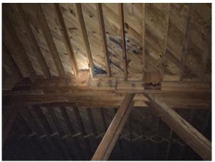
Photo 1: Truss top – signs of water infiltration
