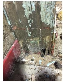
Photo 5: Damaged Column - Hole at Bottom where screwdriver could go in
