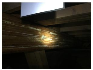
Photo 2: Chord – Potential glue deterioration
