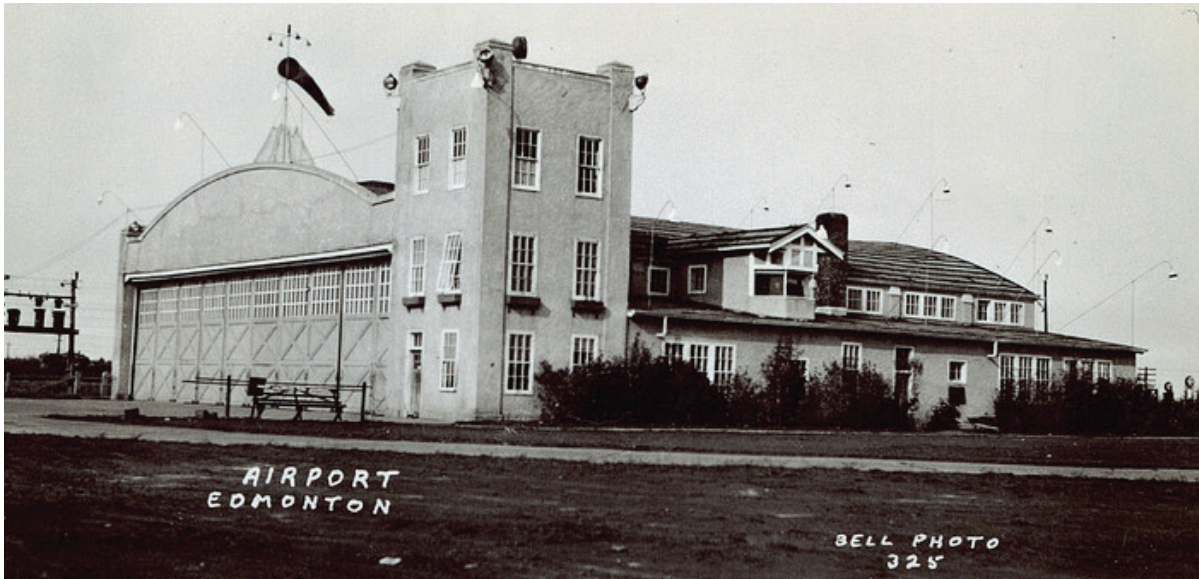
An early photo of the 1929 hangar on the west side of Blatchford Field, built 13 years before the U.S. Army Air Force hangars (including Hangar 11) on the airfield's east side (Peel's Prairie Provinces).
