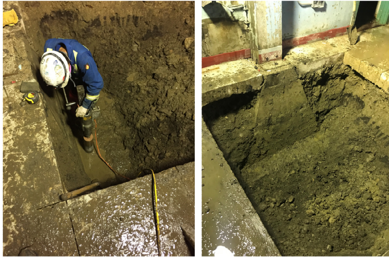
Photos 11 and 12: Foundation Testing and Exposed Foundation
