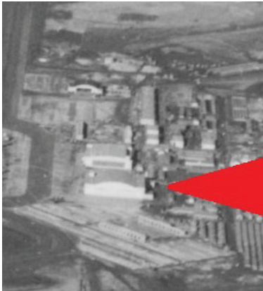
A 1943 photo shows Hangars T2 and T3 constructed, and the office wings for Hangars T1 and T4 already in place. Hangar T3 (Hangar 11) is indicated with a red arrow. (City of Edmonton).
