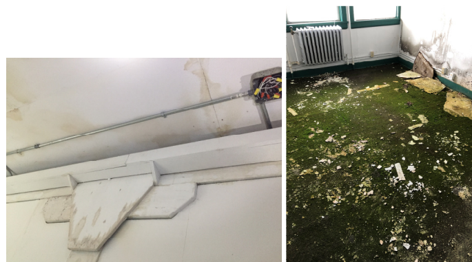
Photos 6 to 7: Ancillary Framing
