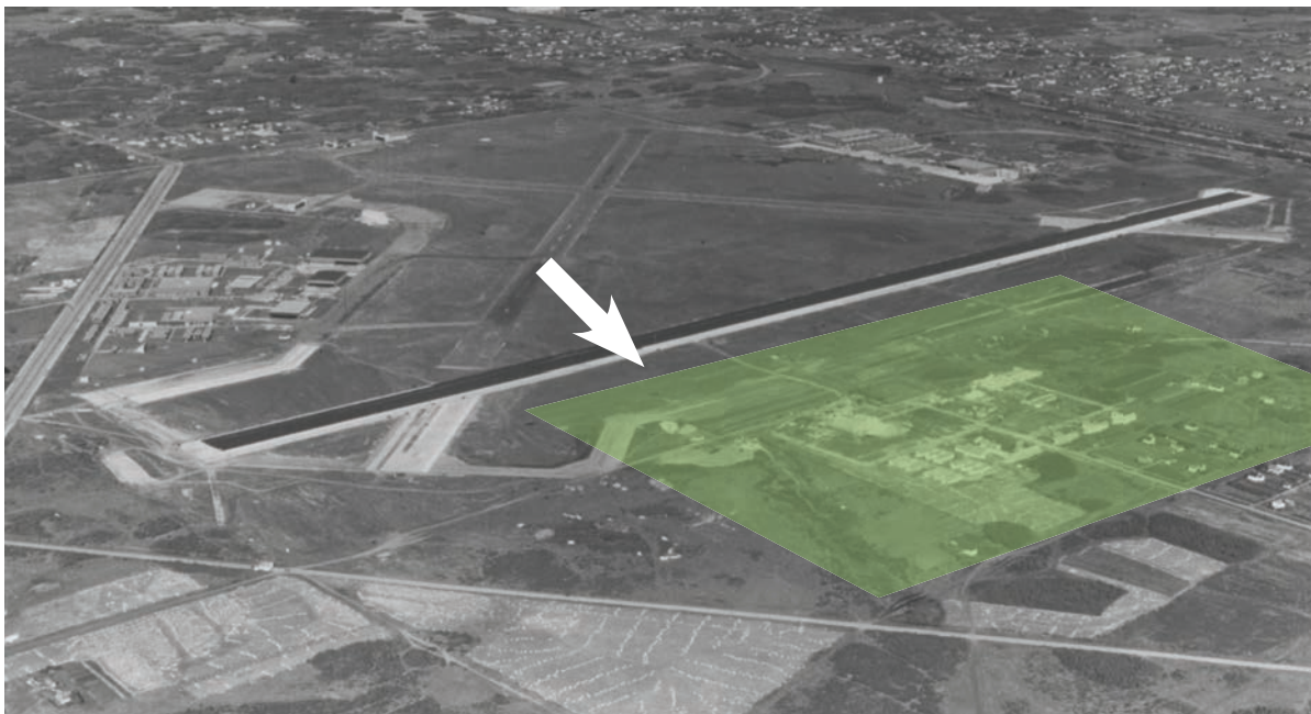
A 1942 photograph shows the general future site of the American detachment (highlighted in green) with only the first few buildings constructed. The future site of Hangar 11 is indicated with a white arrow (City of Edmonton Archives, annotated by ERA).
