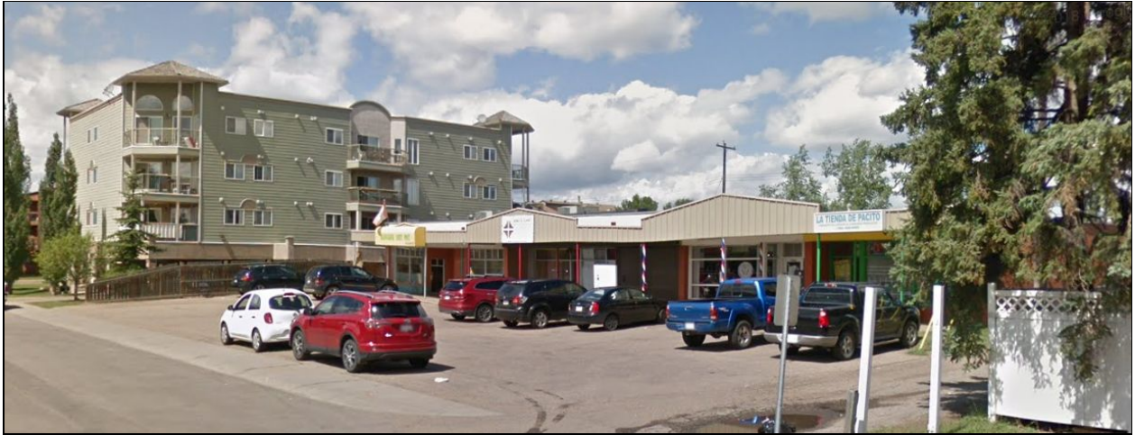
VIEW OF THE SITE AND EXISTING BUILDING FROM 112 AVENUE NW, LOOKING NORTHWEST
