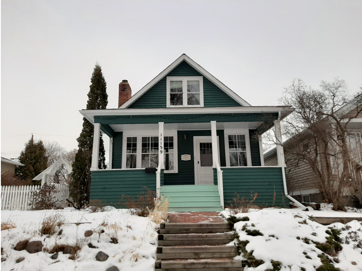
Photo #1 – Front (West) Elevation
