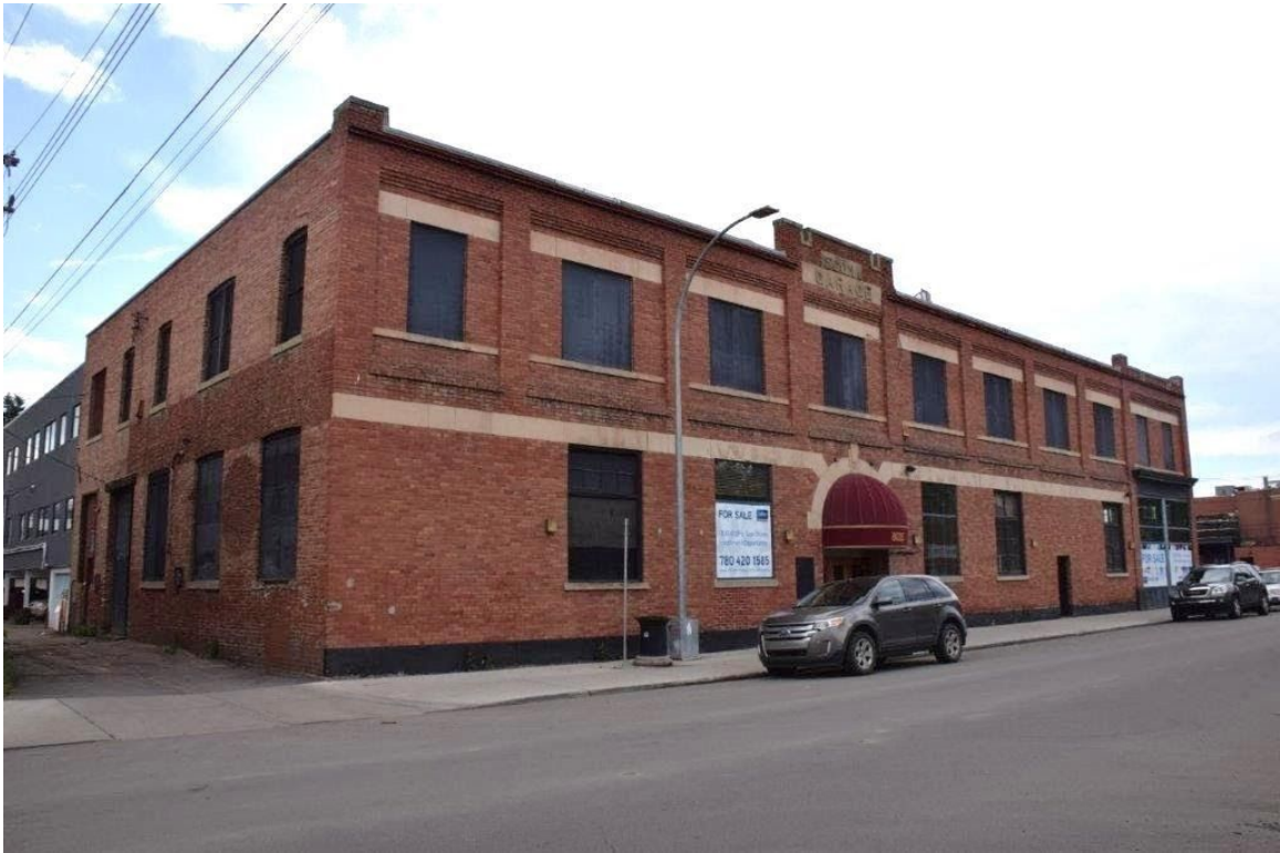
Photo #2 – South and East Façades
