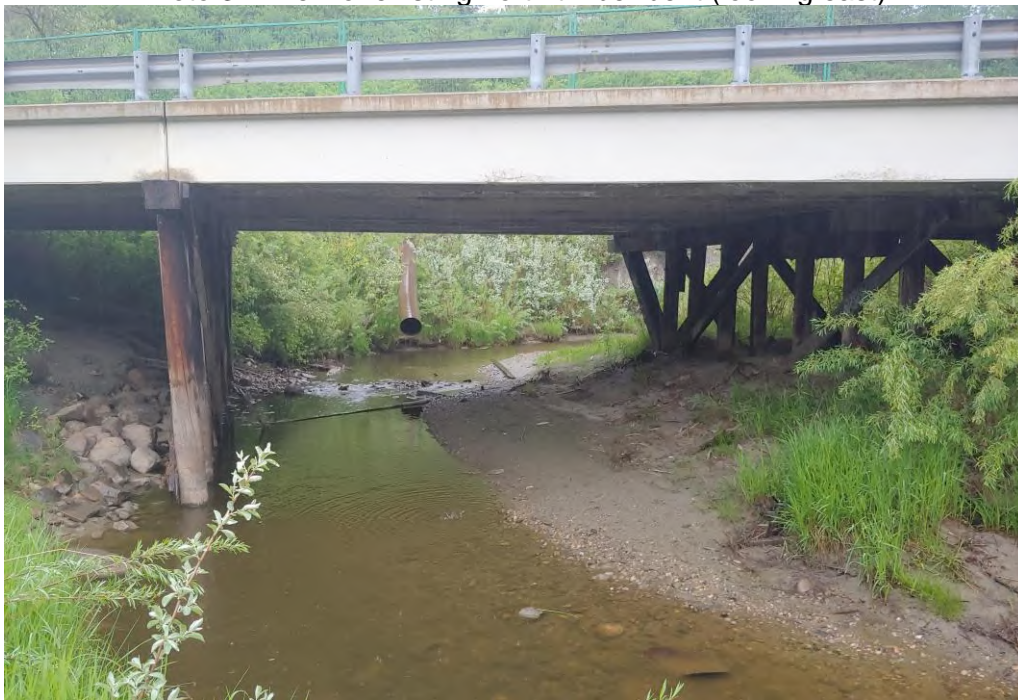
Photo 4 – View of existing timber bents (looking east, upstream).
