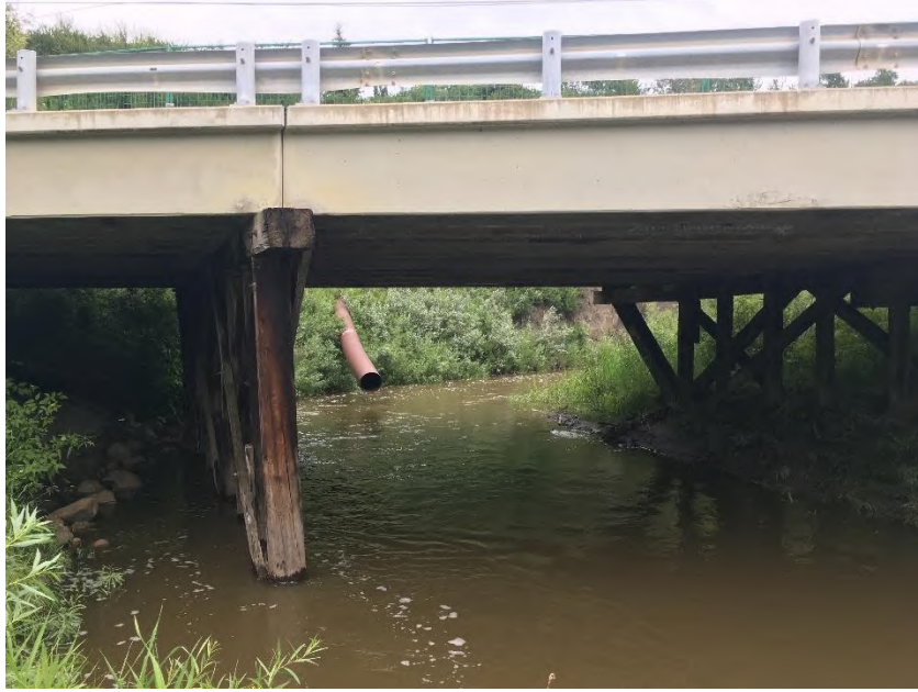
Plate 1.2. Upstream view of Blackmud Creek and treated timber pilings under the pedestrian bridge and culvert pipe out of bank (24 July 2019).
