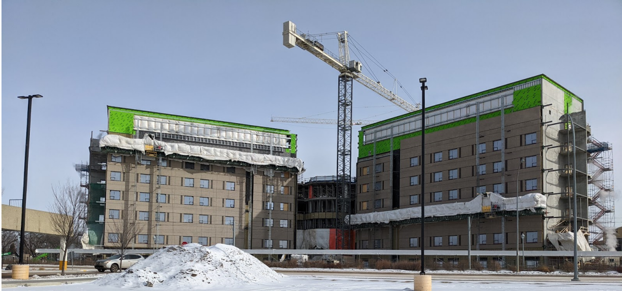
Photo of the site from the west
