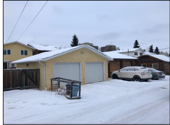
SITE LOOKING NORTHEAST FROM REAR LANE
