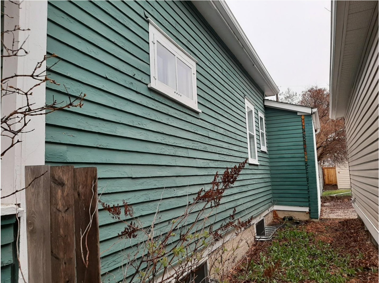
Photo #4 – Side (South) Elevation
