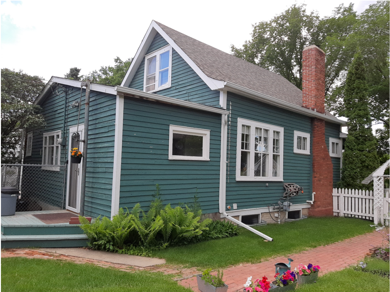
Photo #2 – Rear (West) and Side (North) Elevation
