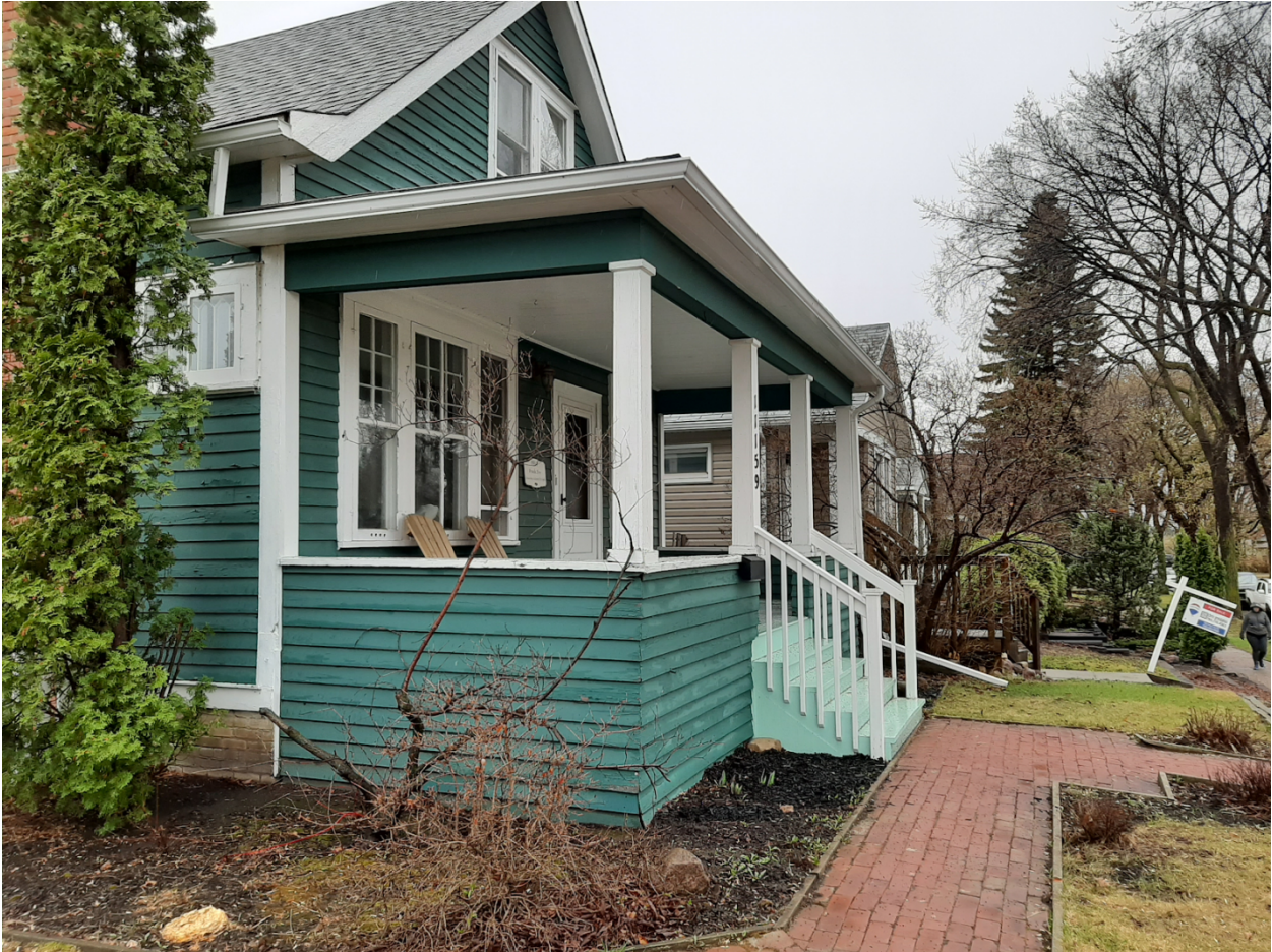
Photo #3 – Side (North) and Front (West) Elevations
