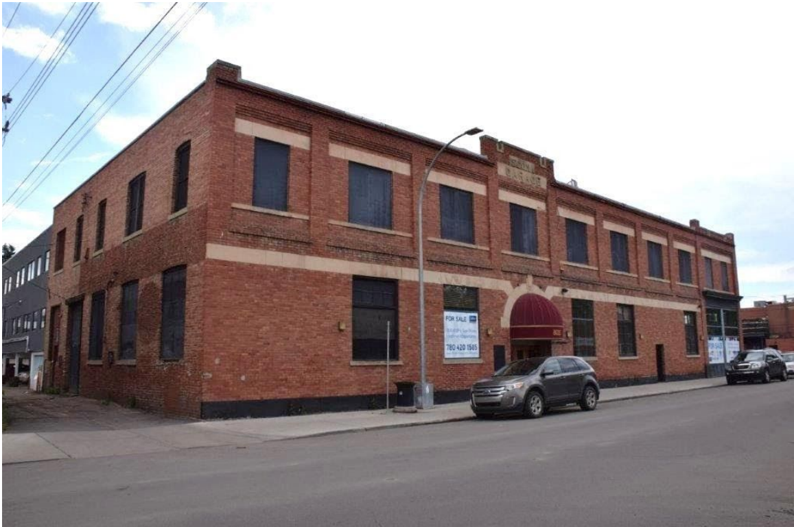
Photo #2 – South and East Façades
