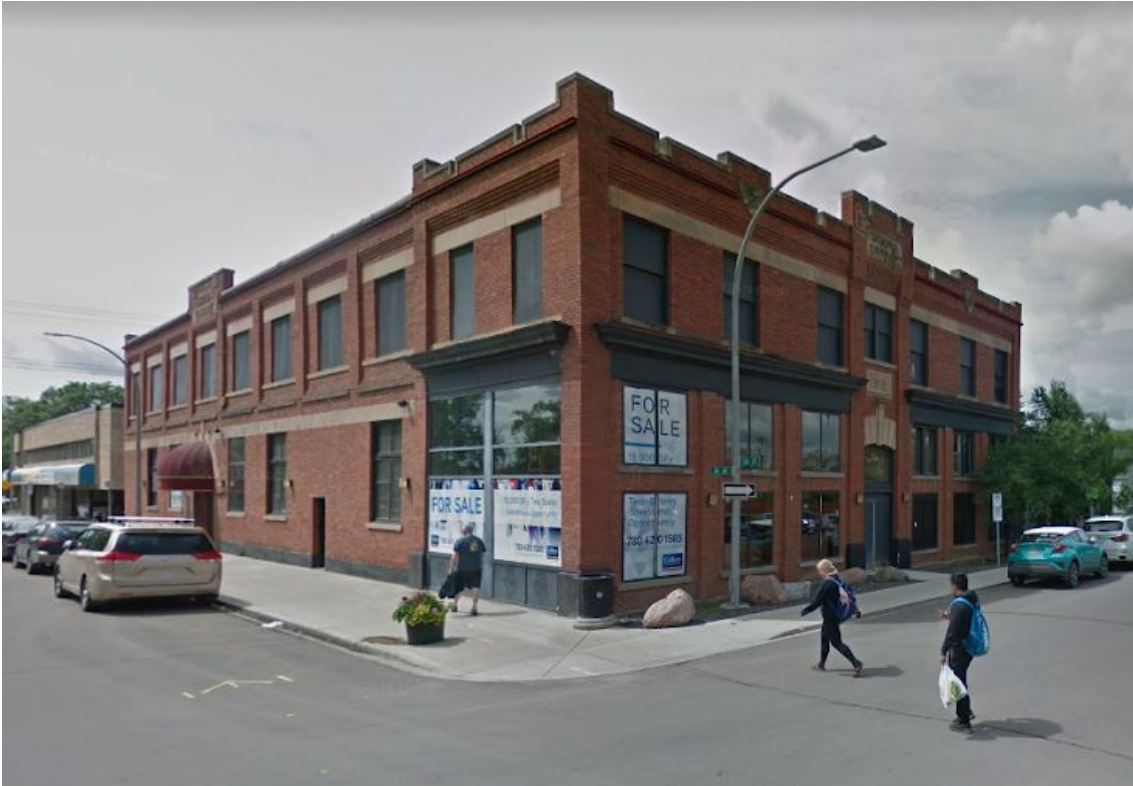
Photo #3 – North and East Façades
