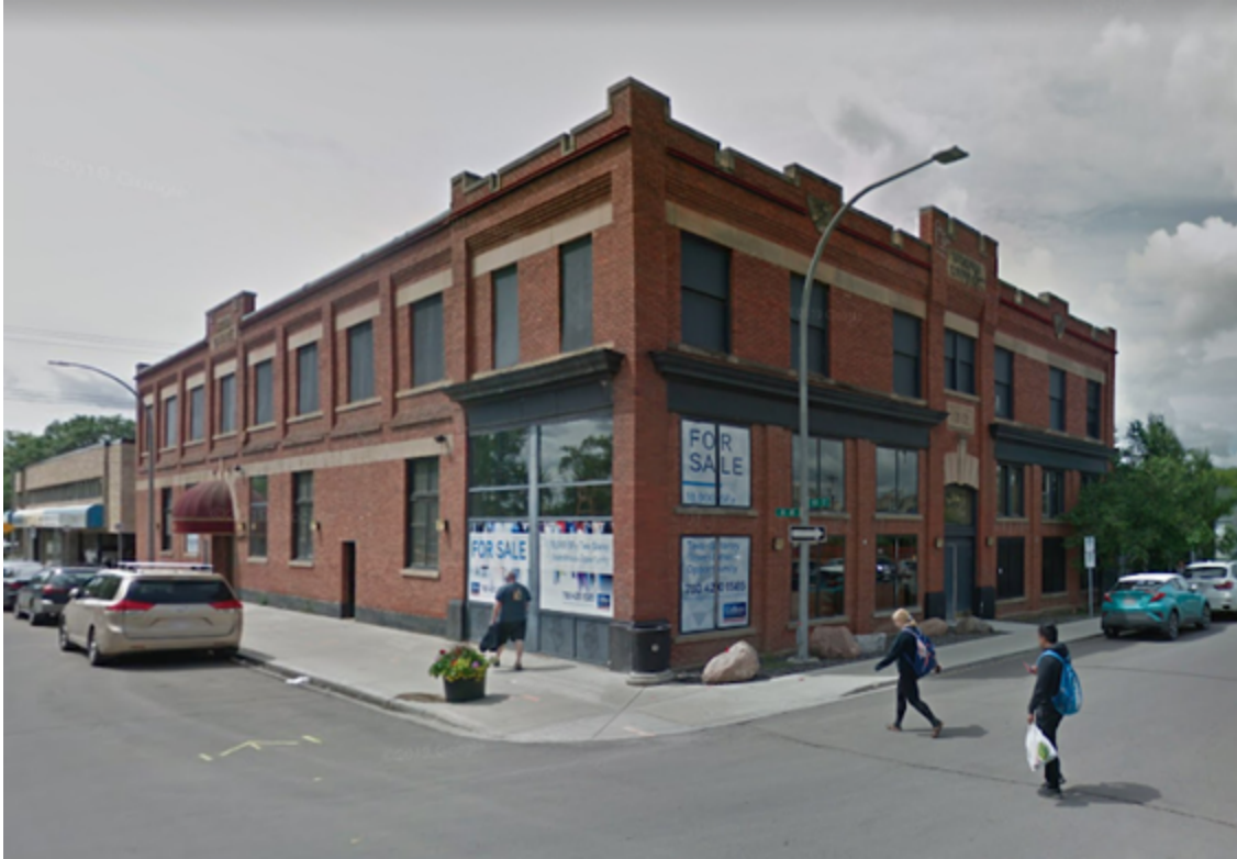
North and East Facades
