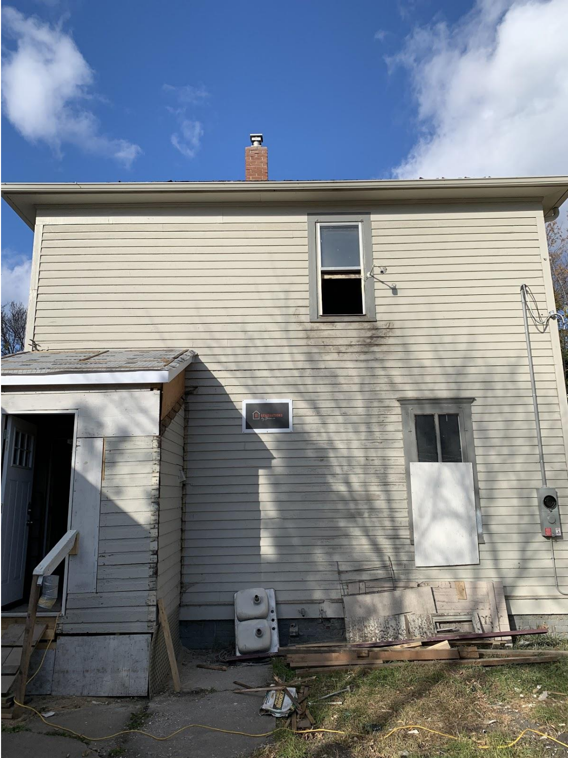
Photo #2 – Rear (South) Elevation
