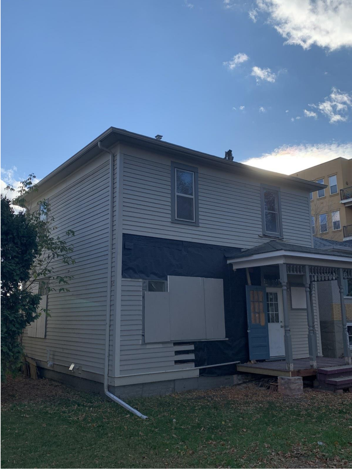
Photo #3 – Side (East) and Front (North) Elevations
