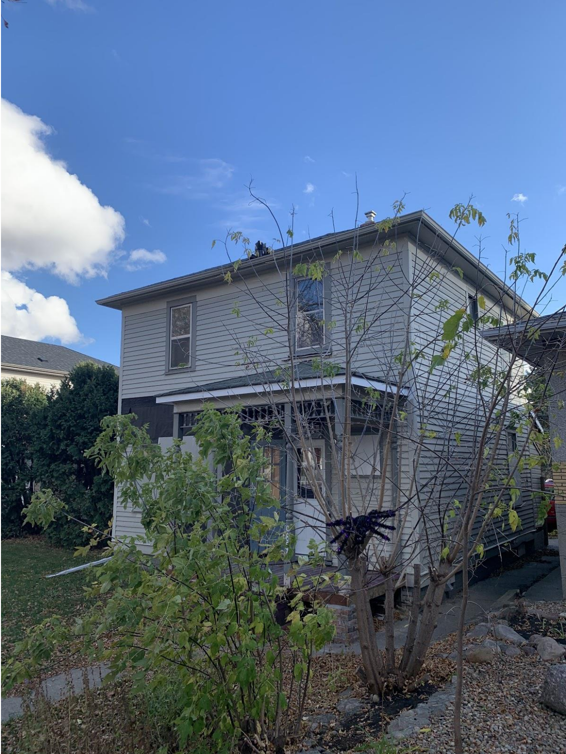
Photo #4 – Side (West) and Front (North) Elevations
