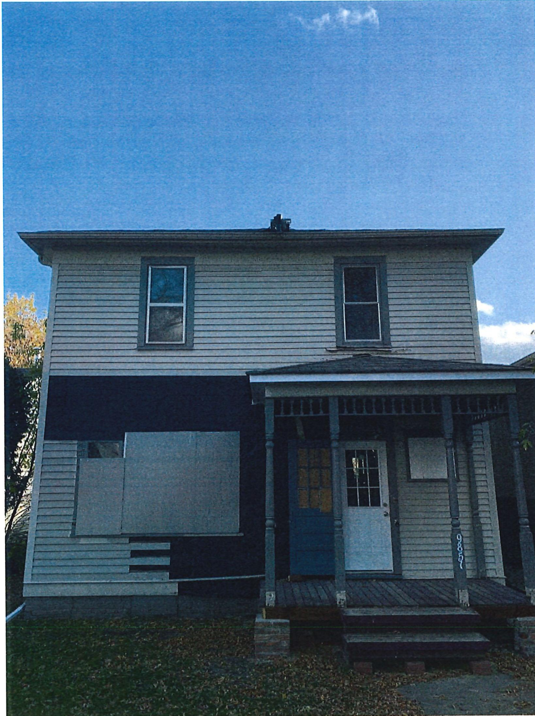
Photo #1 – Front (North) Elevation
