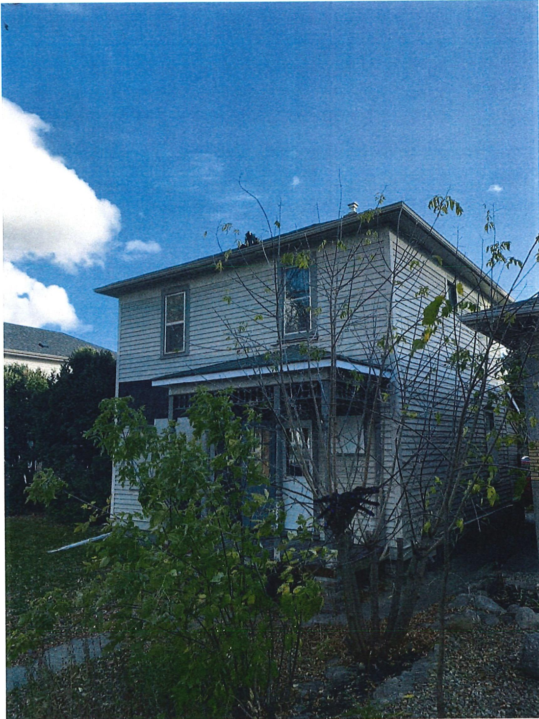
Photo #4 – Side (West) and Front (North) Elevations
