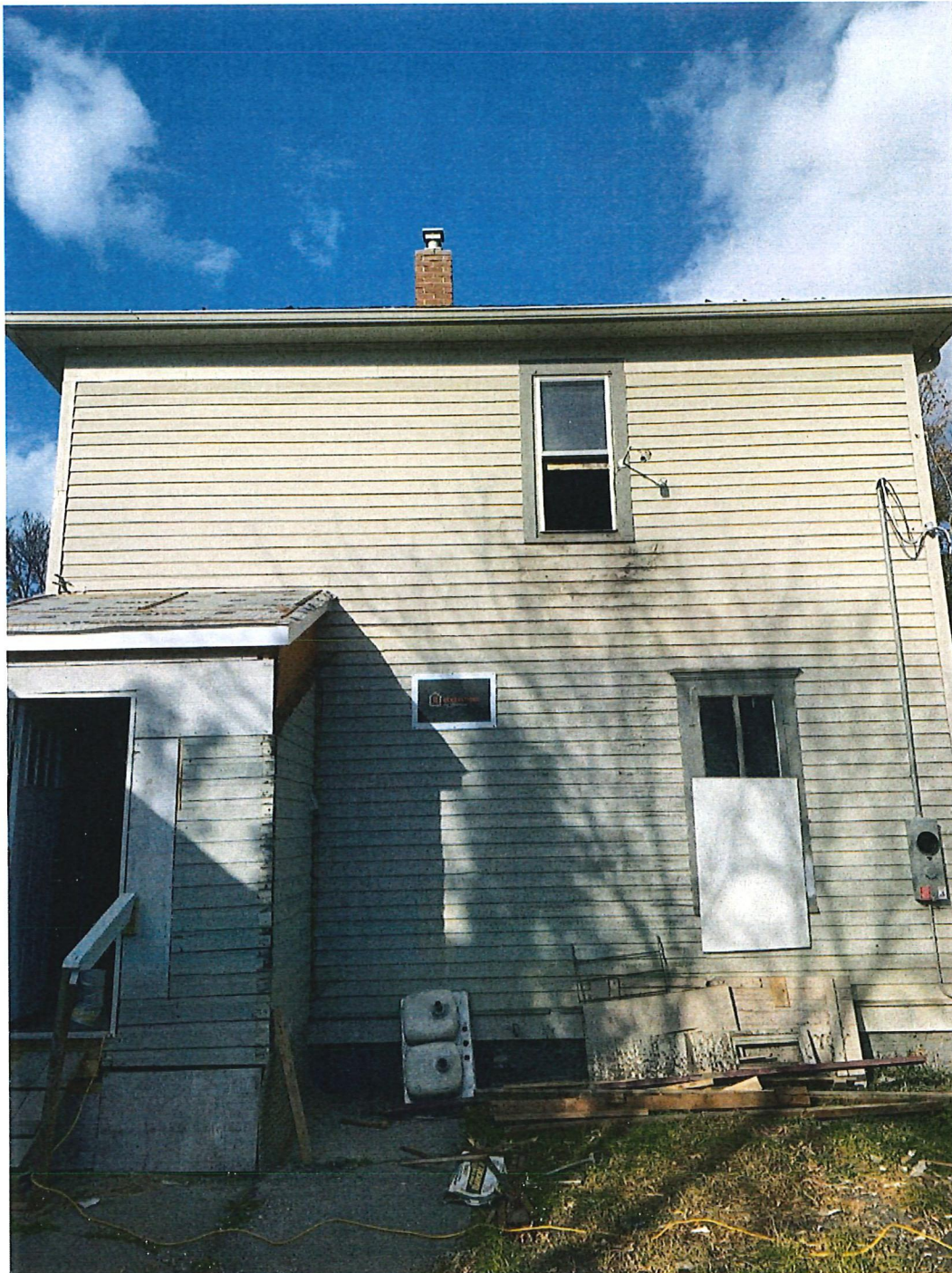
Photo #2 – Rear (South) Elevation
