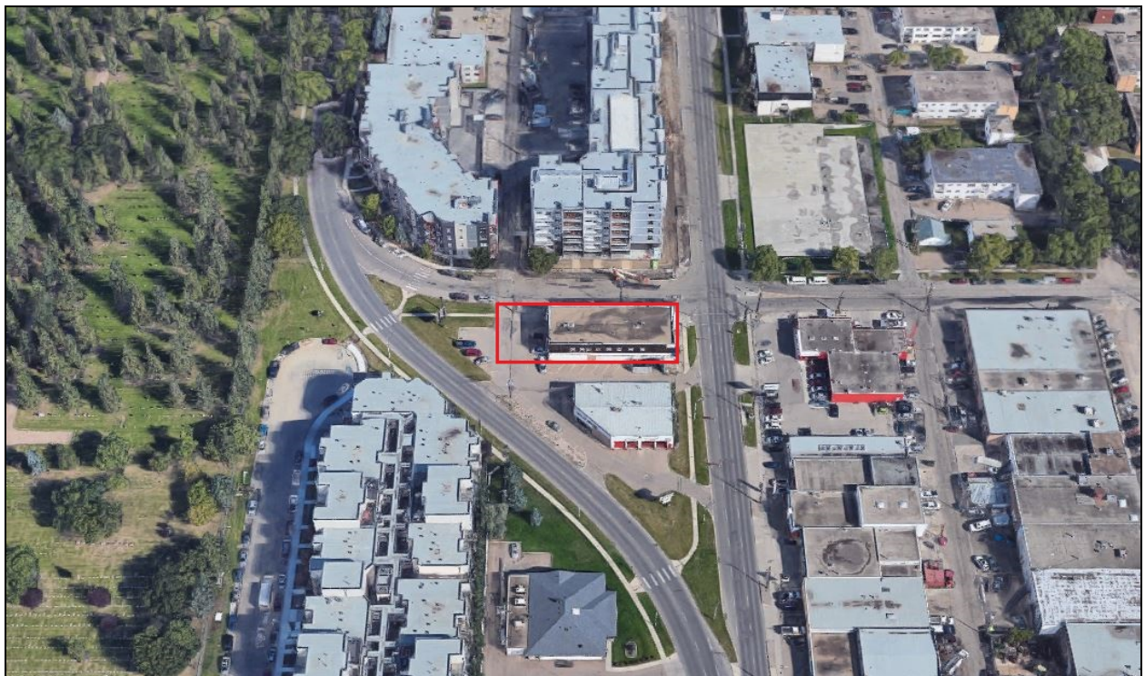
AERIAL VIEW OF EXISTING COMMERCIAL BUILDING FROM THE SOUTH
