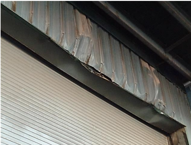
View of damaged metal cladding at overhead doors on the west elevation of the Tipping Building
