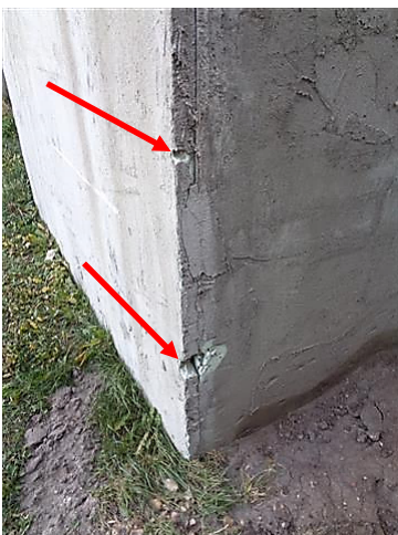
View of damaged foundation insulation and parging on the southwest corner of the Tipping Building
