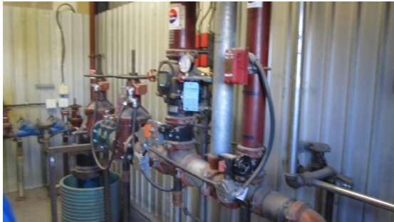
Typical view Service room #2 sprinkler tree
