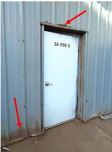
View of corrosion on metal cladding on the south elevation of the Finishing Building
