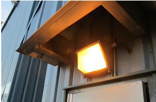
Typical exterior fixture with HID sodium Lamp
