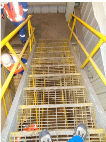
View of typical metal-framed stairs in Dewatering Building stairwell
