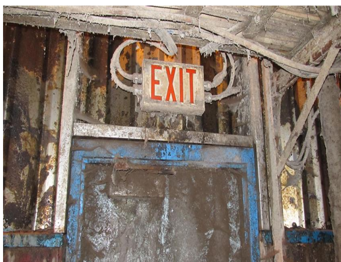
South Download Pull-station requiring cleaning Finishing Building typical exit sign requiring cleaning
