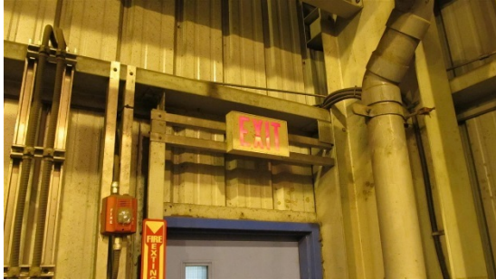
View of Dewater Building, typical interior roof rain leaders View of typical interior roof rain leaders
