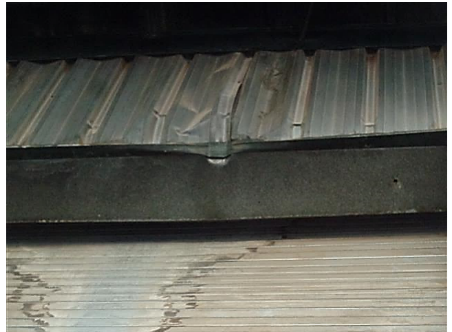
View of damaged metal cladding at overhead doors on the west elevation of the Tipping Building
