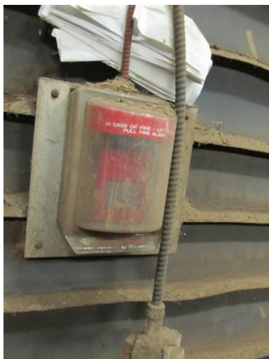
South Download Pull-station requiring cleaning Finishing Building typical exit sign requiring cleaning
