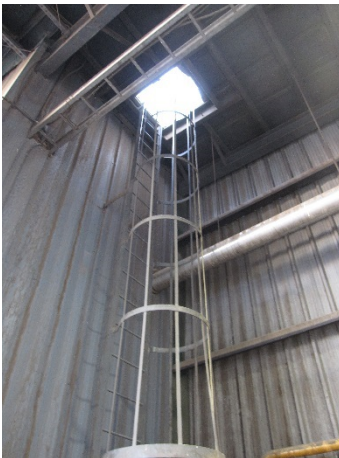
View of roof access ship ladder on the northwest corner of the Tipping Building
