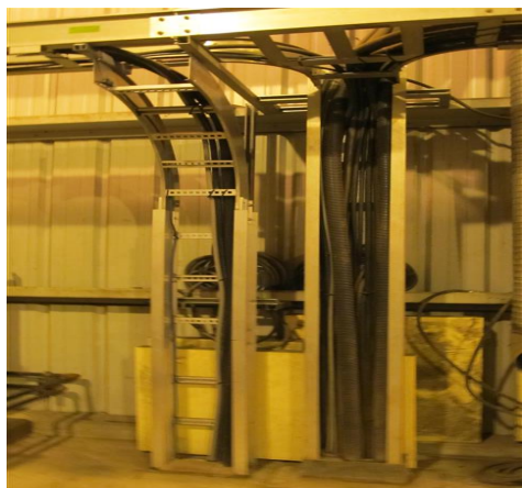
Dewater Building cable tray system
