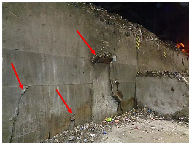
View of typical damaged and torn metal plating on the push wall in the tipping area.
