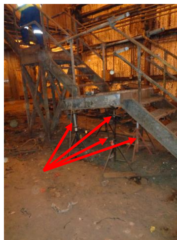
View of metal-framed stairs leading to electrical room mezzanine within the North Download Building with temporary supports
