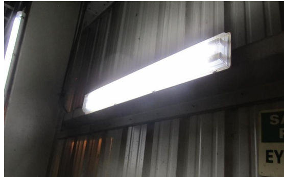
Typical dust proof fluorescent two lamp T8 fixture
