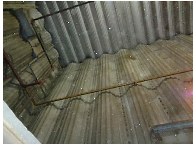
View of typical metal panel liner on the interior of the Finishing Building
