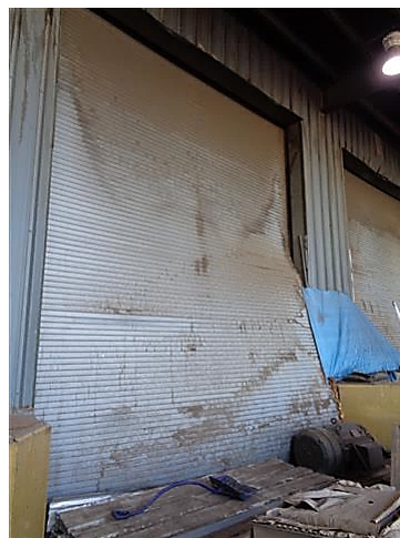
View of non-functioning damage to overhead doors on the west elevation of the Tipping Building
