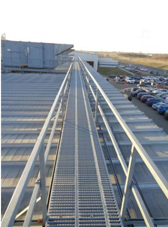
View of typical Fall Protection guard rails and maintenance walkways on the roof of the Tipping Building
