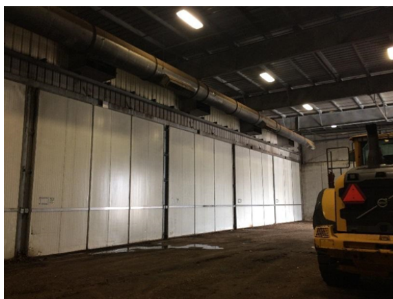
Figure 3-3 Air-tight Door on the Outside of Composting Tunnels
