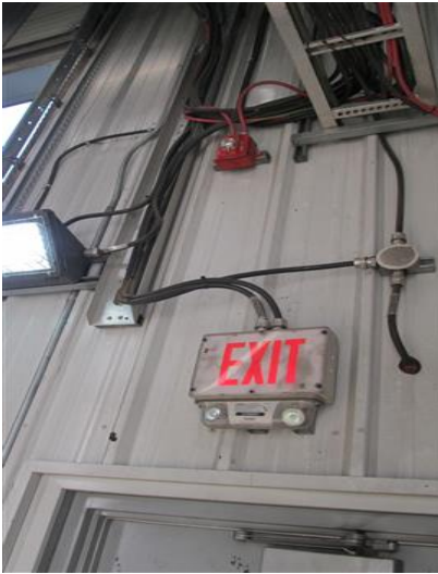
Typical Exit/EM light over egress exit
