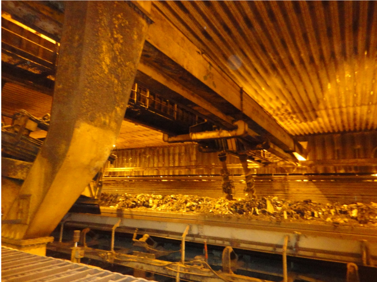
Picture 3-3 - Turner assembly showing the rotating screws (right), bridge (top) and conveyor track (bottom left)
