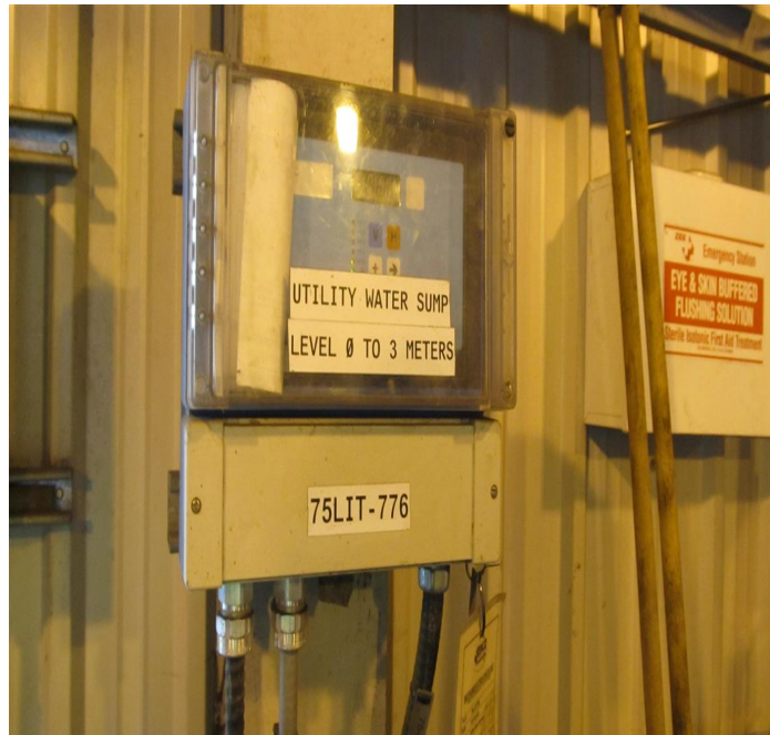
Controller for Sump Pump in Pump Building to lagoon
