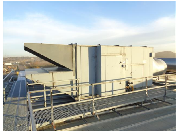
View of typical Fall Protection guard rails and maintenance walkways on the roof of the Tipping Building
