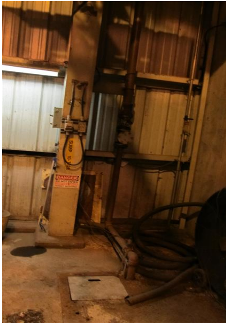
Typical Sump Pump Dewater Building
