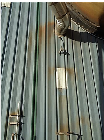
View of damaged metal cladding at overhead doors on the west elevation of the Tipping Building
