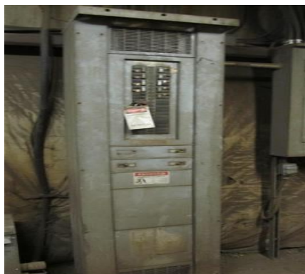
Panelboard 20-PNL-2B Tipping Floor
