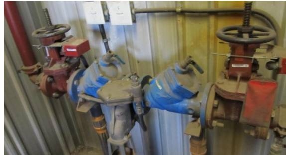
Typical view of Back-Flow Prevention Device
