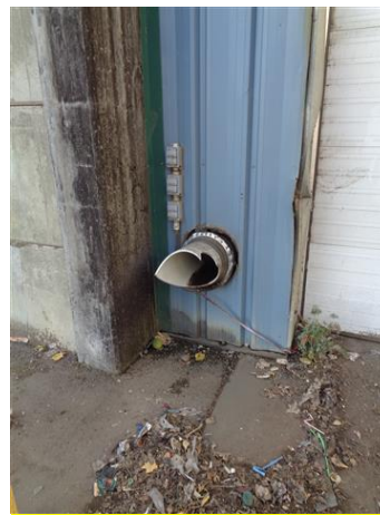
View of damaged rain leader on the east corner of the Tipping Building
