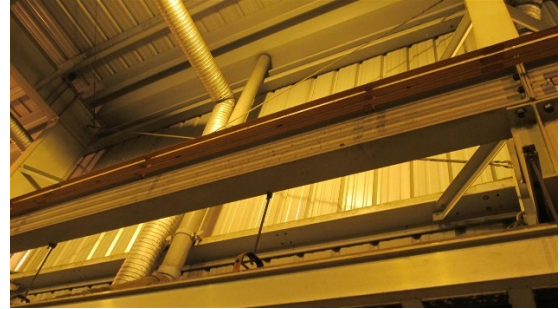
View of Dewater Building, typical interior roof rain leaders View of typical interior roof rain leaders
