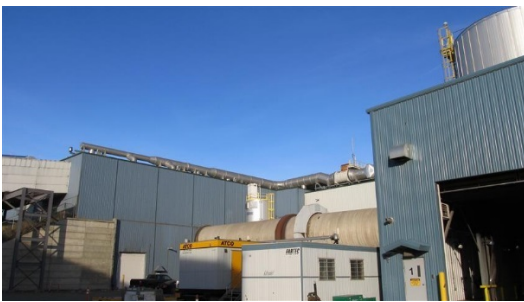
Roof mounted exhaust ducting Tipping Building
